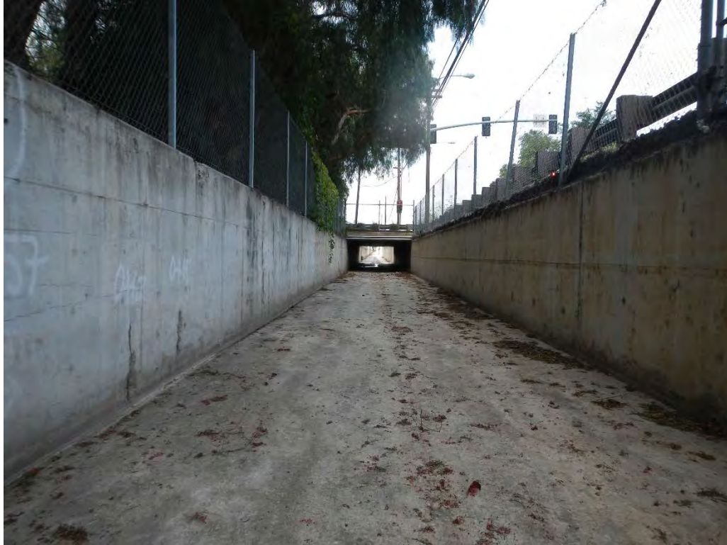
FIGURE A-13. LOOKING DOWNSTREAM TOWARDS VISTA ARROYO DR./ANDALUSIA DR. CROSSING
