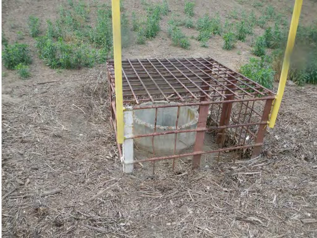
FIGURE A-3. PRIMARY SPILLWAY ENTRANCE W/ TRASH RACK
