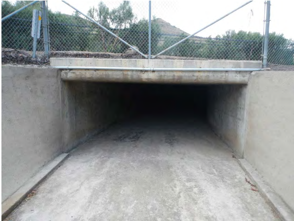
FIGURE A-11. UPSTREAM FACE OF SANTA ROSA ROAD CULVERT, LOOKING DOWNSTREAM
