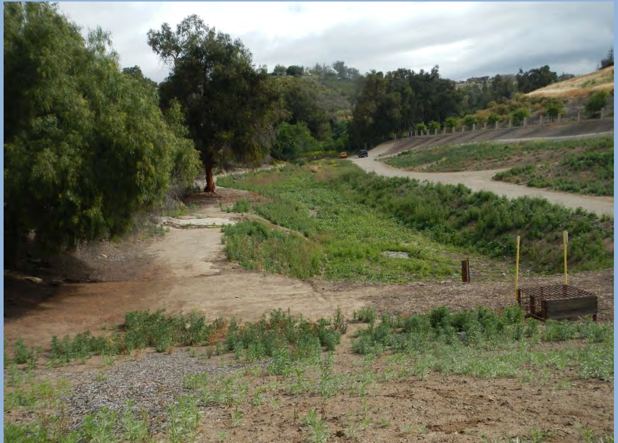
Photo: Santa Rosa Road No. 2 Debris Basin, looking upstream from crest
