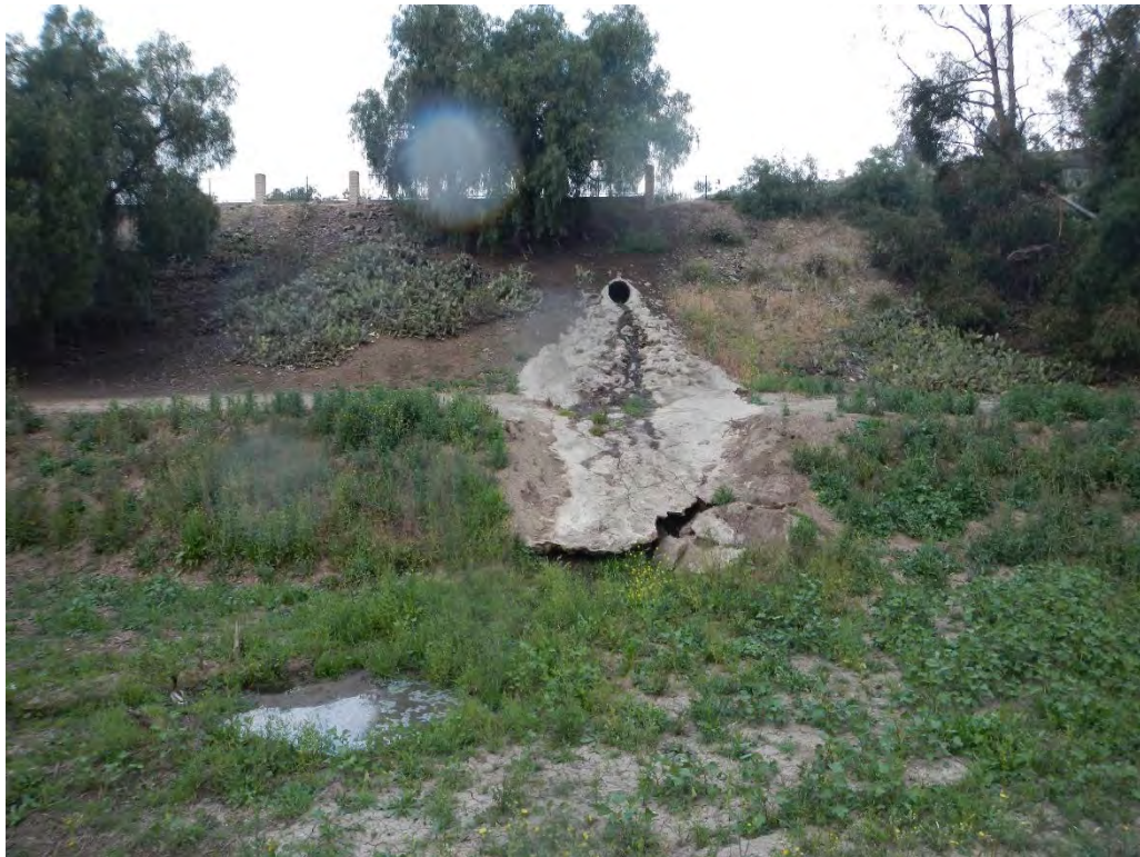
FIGURE A-2. DOWNSTREAM DAM FACE, PRIMARY SPILLWAY OUTLET
