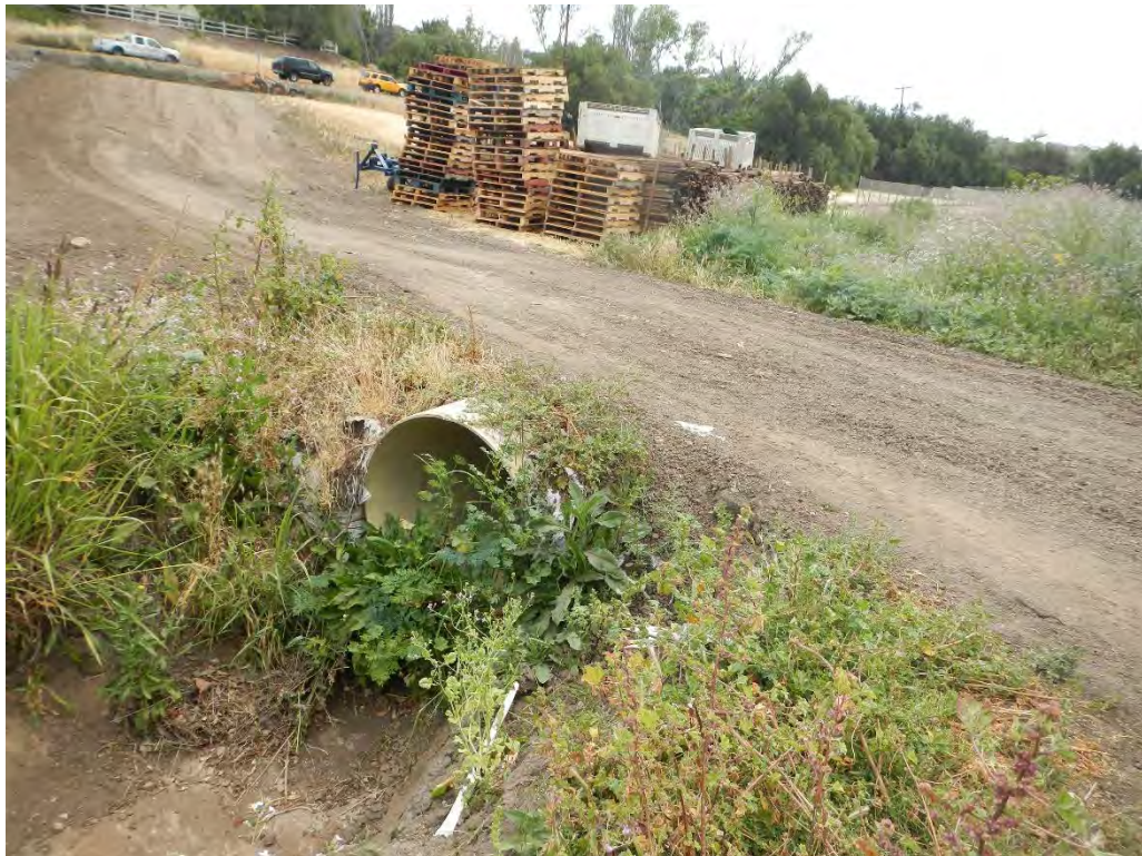
FIGURE A-14. UN-NAMED FARM ROAD CULVERT CROSSING
