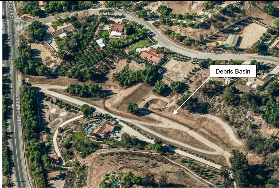
a. Oblique view of the No. 2 Debris Basin
