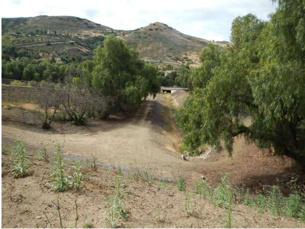
FIGURE A-9. DOWNSTREAM CHANNEL, EMERGENCY SPILLWAY EXIT ON LEFT
