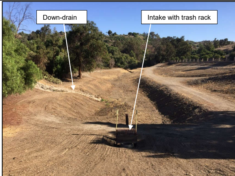
b. No. 2 Debris Basin from the dam crest, facing north
