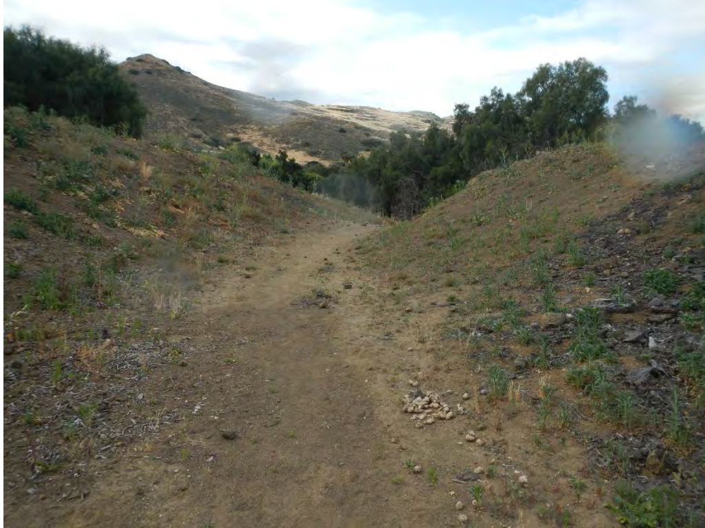
FIGURE A-7. EMERGENCY SPILLWAY ENTRANCE, LOOKING DOWNSTREAM
