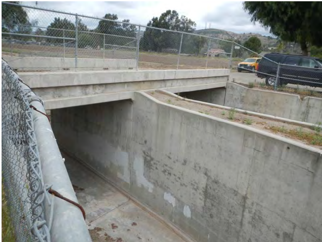
FIGURE A-18. CULVERT AT DOWNSTREAM CONFLUENCE WITH CONEJO CREEK
