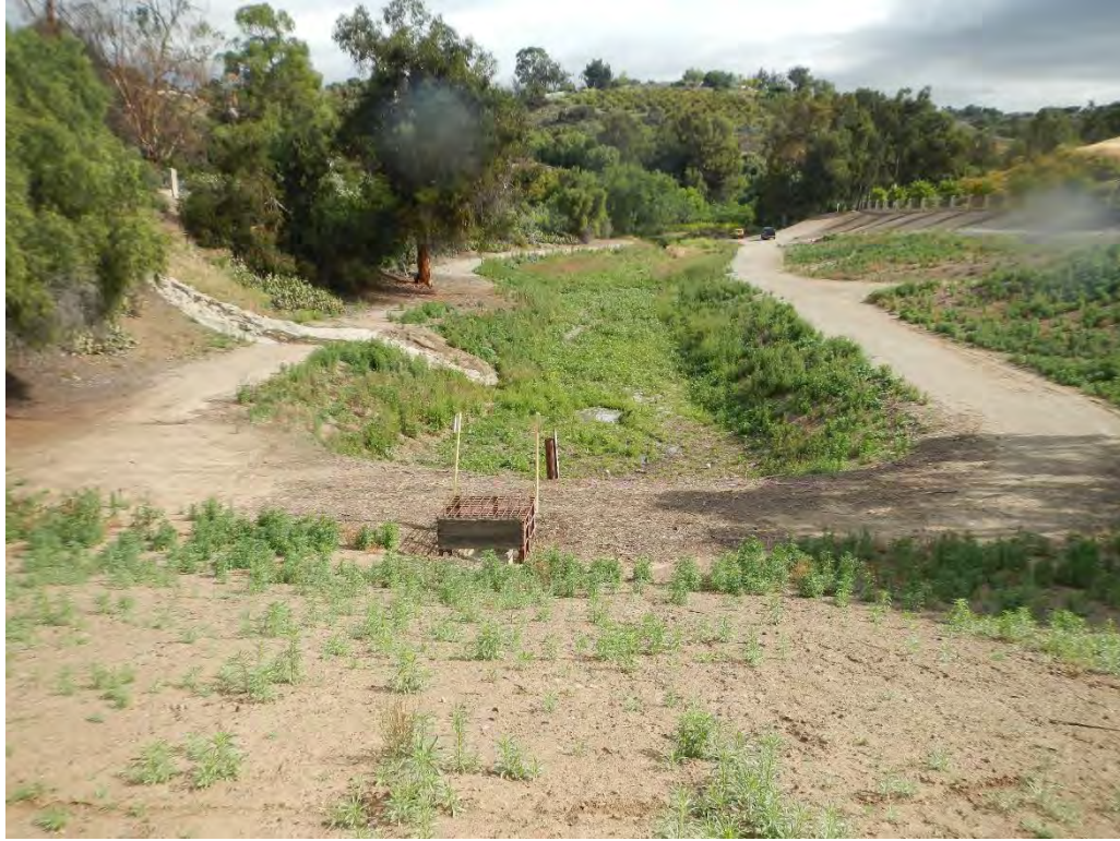
FIGURE A-5. DEBRIS BASIN, LOOKING UPSTREAM FROM TOP OF DAM
