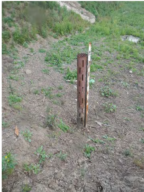
FIGURE A-4. DEBRIS BLEEDER/RISER PIPE AT BOTTOM OF UPSTREAM DAM FACE
