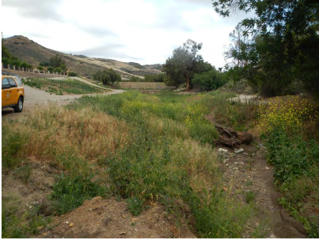
FIGURE A-1. DEBRIS BASIN AND UPSTREAM DAM FACE
