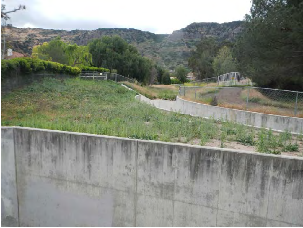
FIGURE A-17. DOWNSTREAM CONFLUENCE WITH CONEJO CREEK
