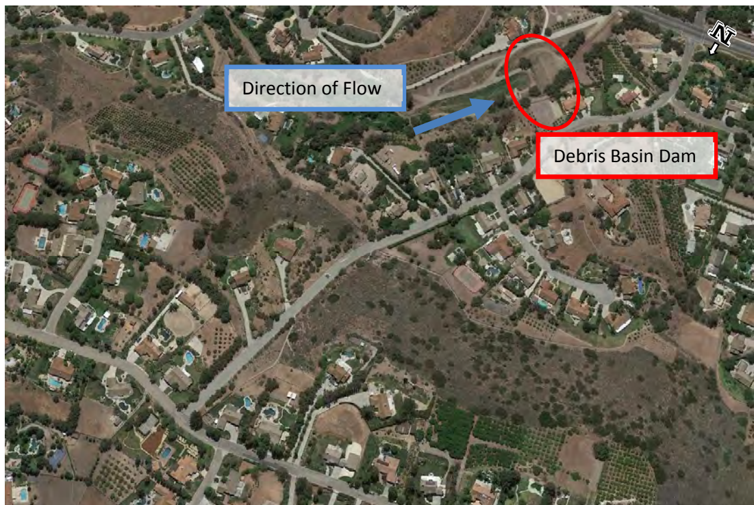
Figure 2-9. Debris Basin Aerial Photo, 2015
