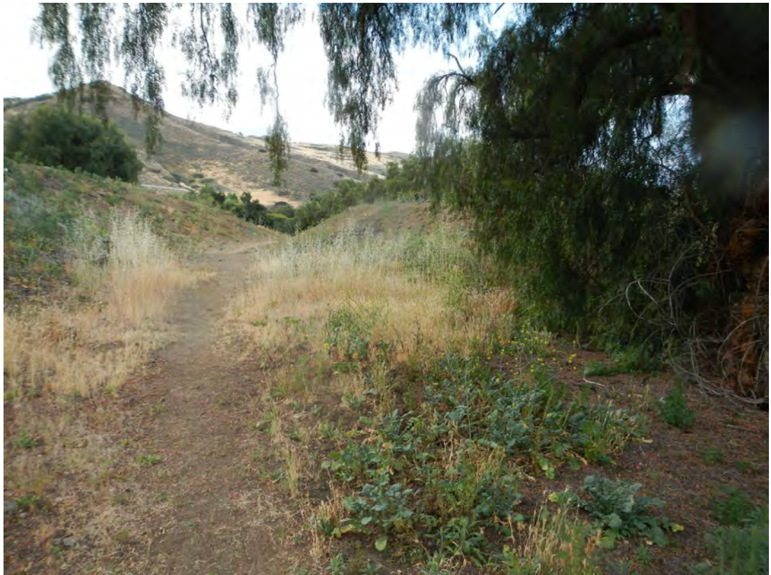
Figure 2-3. Emergency Spillway, Looking Downstream
