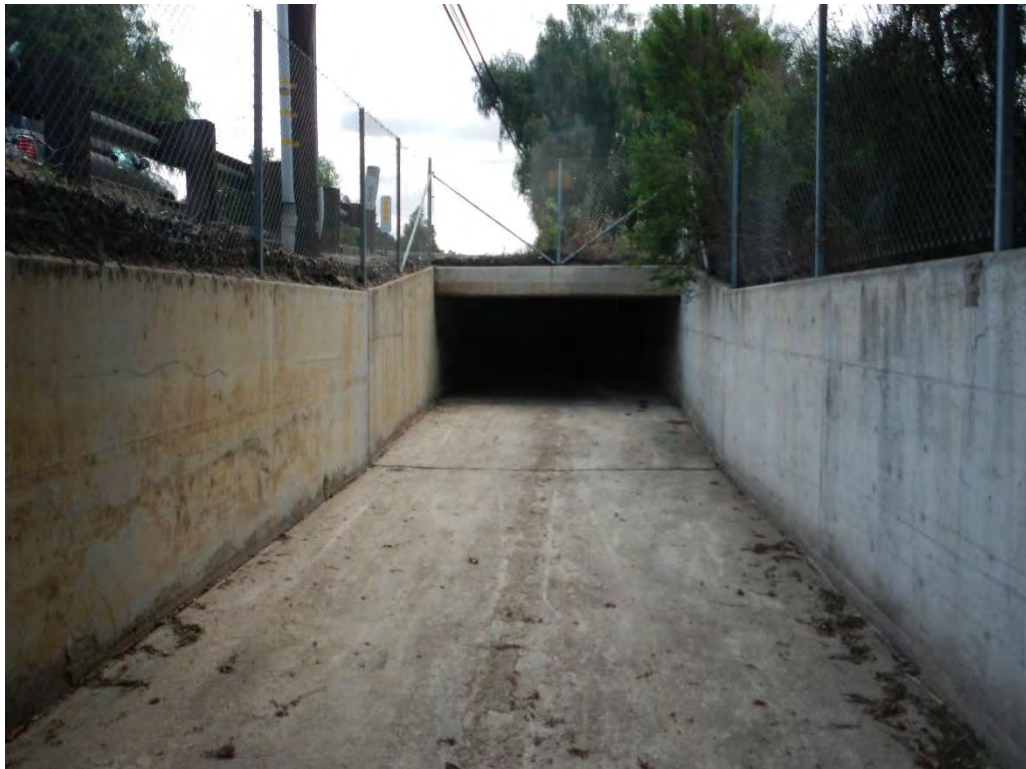
FIGURE A-12. DOWNSTREAM FACE OF SANTA ROSA ROAD, LOOKING UPSTREAM
