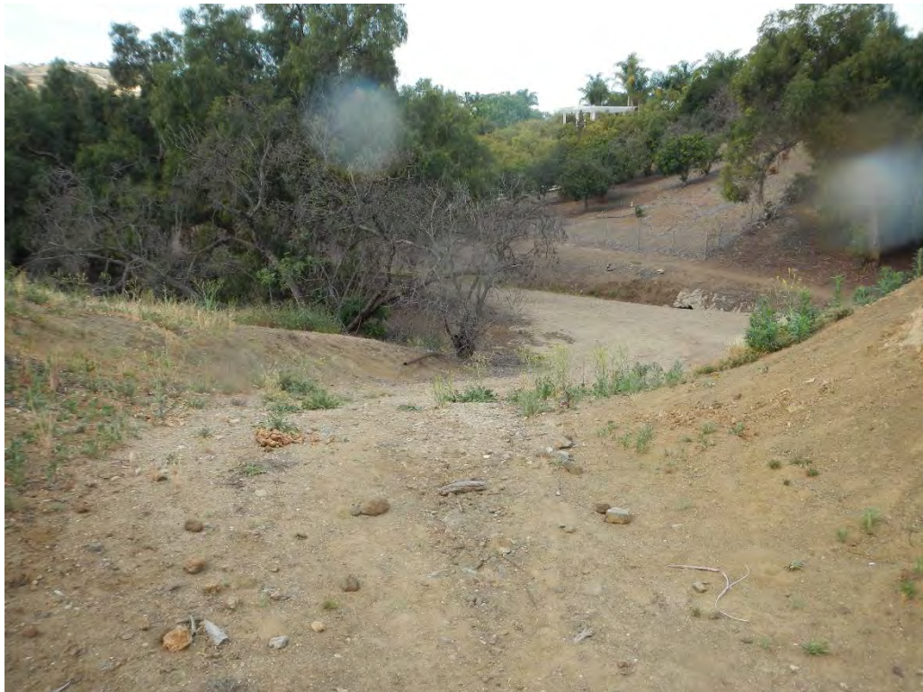
FIGURE A-8. EMERGENCY SPILLWAY, LOOKING DOWNSTREAM AT CHANNEL JUNCTION
