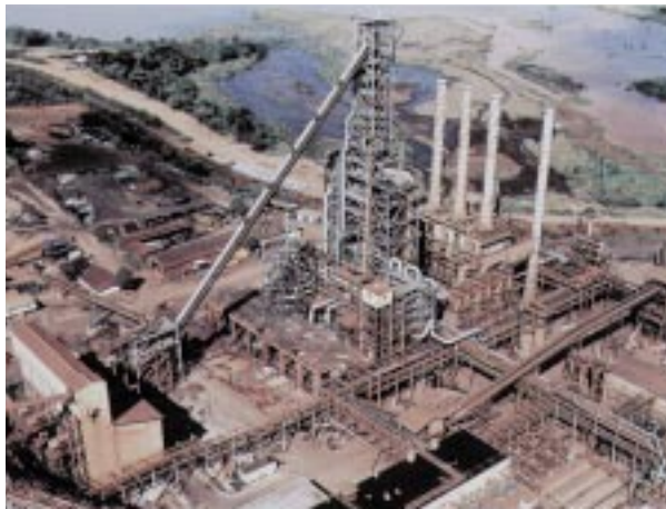
Hot briquetted iron plant of Operaciones al Sur del Orinoco (OPCO), a company in Puerto Ordaz, Venezuela
