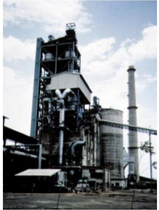
Chinfon Cement Factory, under construction in Vietnam
