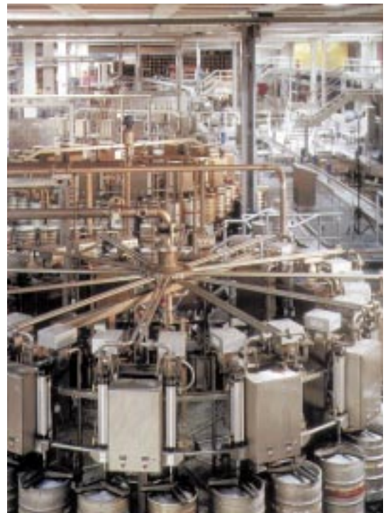
Cleaning and filling facility manufactured by Till GmbH of Germany
