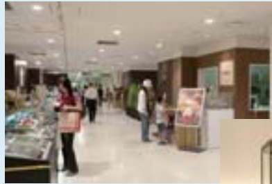
Construction to even out the floor on the food hall has been progressing smoothly since August 2005
