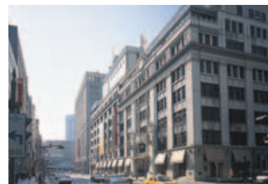
Mitsukoshi Nihonbashi main store
