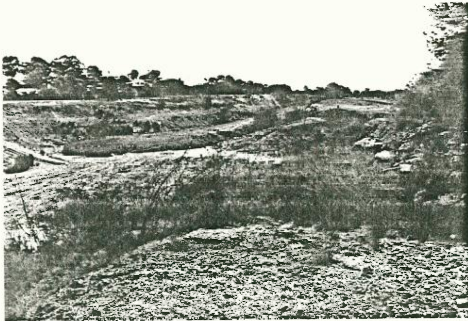
CURRENT INFILLING OF PART OF THE SITE WITH PELTON COLLIERY'S WASHERY REJECT MATERIAL.
