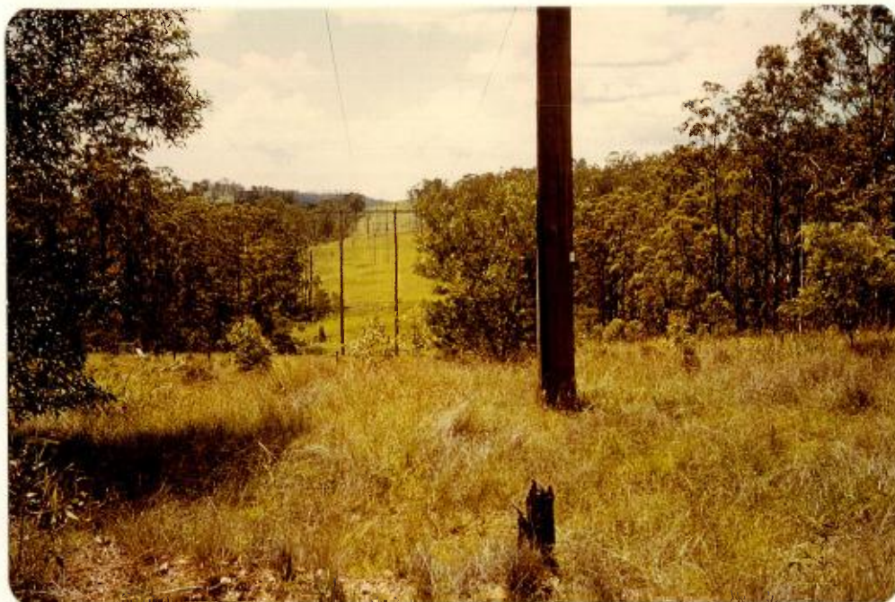
PLATE 6 Land clearing for power-line easement close to Drake.
