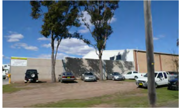
Photo 3 - Poor example of blank wall treatment
