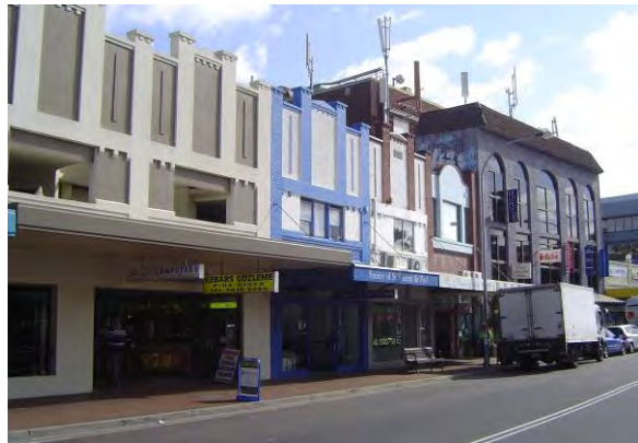
Photo 2.6: View of existing buildings along Longueville Road
