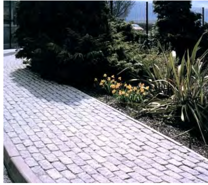
Photo 6 - Use of pavers for pathway treatment to blend in with landscape of the dwelling.
