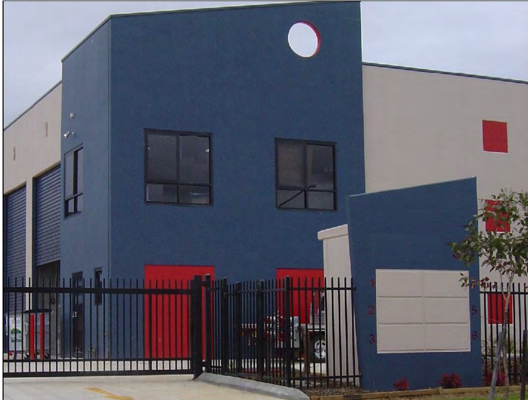
Figure 3 Character of Industrial Buildings
