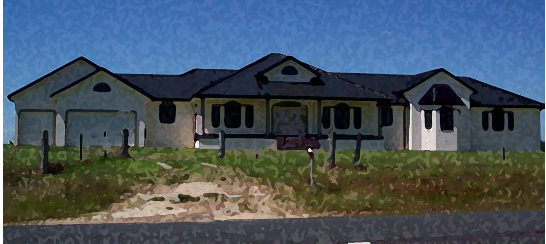
Figure 1 Poor location of building
