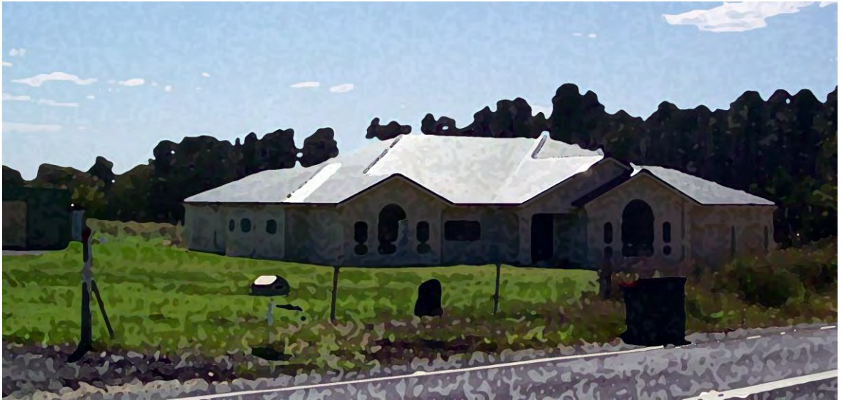
Figure 7 Poor example of Streetscape
