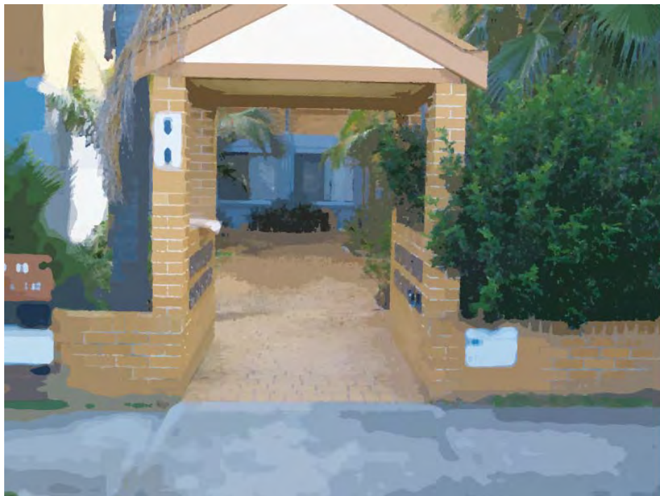
Figure 7 Entry to the Residential Flat Building
