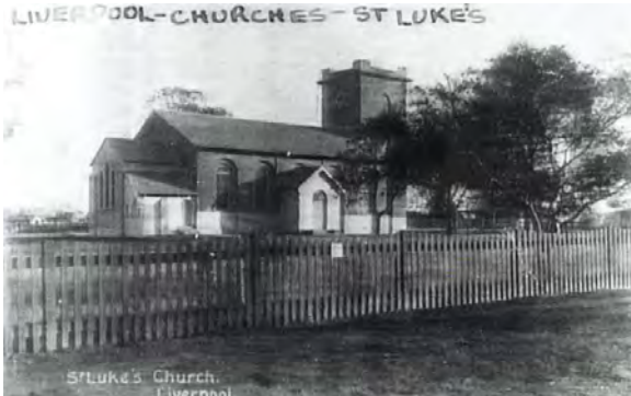
Figure 27 St Luke's Church
