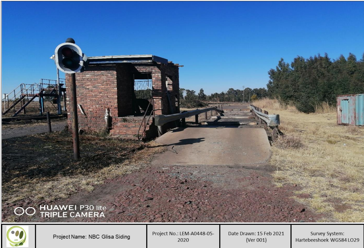
Figure 3: Existing Weighbridge and office to be refurbished.
