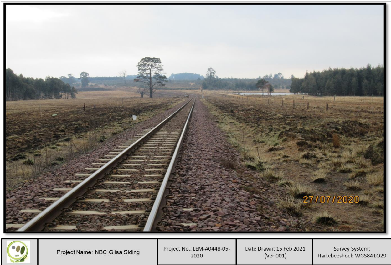
Figure 2: Existing Railway at Glisa Siding to be refurbished.
