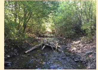
Planebed channel post-restoration
