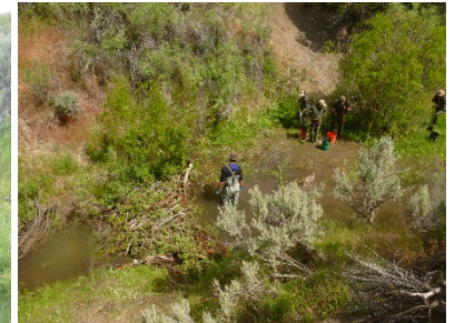
Left: BDA complex built using posts and willow weave Right: Postless BDA built using juniper
