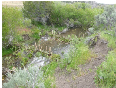
Left: BDA complex built using posts and willow weave Right: Postless BDA built using juniper
