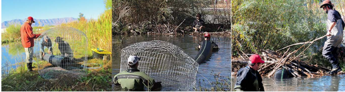
Figure 14 – Pond leveler installation. From left: securing flexible pipe in cage to protect inflow from being clogged; placing pipe into beaver pond; rebuilding beaver dam after setting pipe into notched dam at desired water height.
