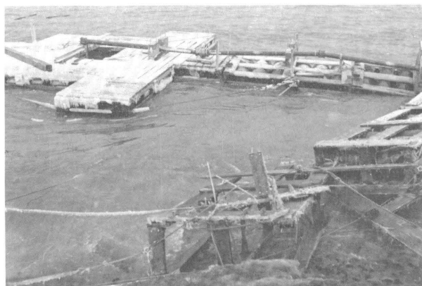
Figure 1. Rafts for saltwater intake were damaged by rough seas.
