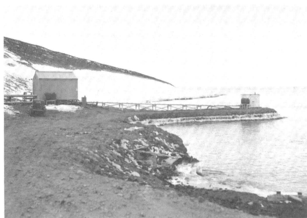
Figure 2. Pump house, heated pipe, and intake house on new jetty.
