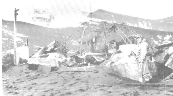
Figure 2. Remains of living hut at Chilean station destroyed by eruption on February 21, 1969. Ash and scoria mantle surface in foreground. Fissure, mostly concealed by steam, lies on far side of bomb-covered slope behind station.
