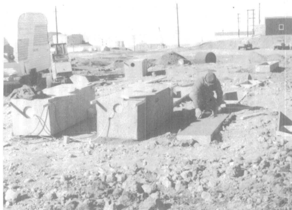
Figure 5. General view of test site. Note protective wooden hoods to permit curing at elevated temperatures.
