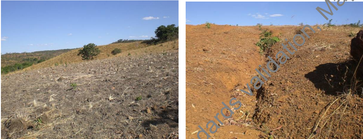
Figure 34: Photo left: plantation area recently prepared using grading (geographic location: 10°15.39' S, 48°07.14' W); Photo right: early stages of gullying, arising from the use of inappropriate soil management techniques (geographic location: 10°14.31' S, 48°07.058' W)
