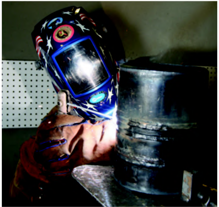
Fig. 5 — Army veteran Kenneth Duvall welds on a section of pipe as part of the VIP accelerated pipe welding training program.
