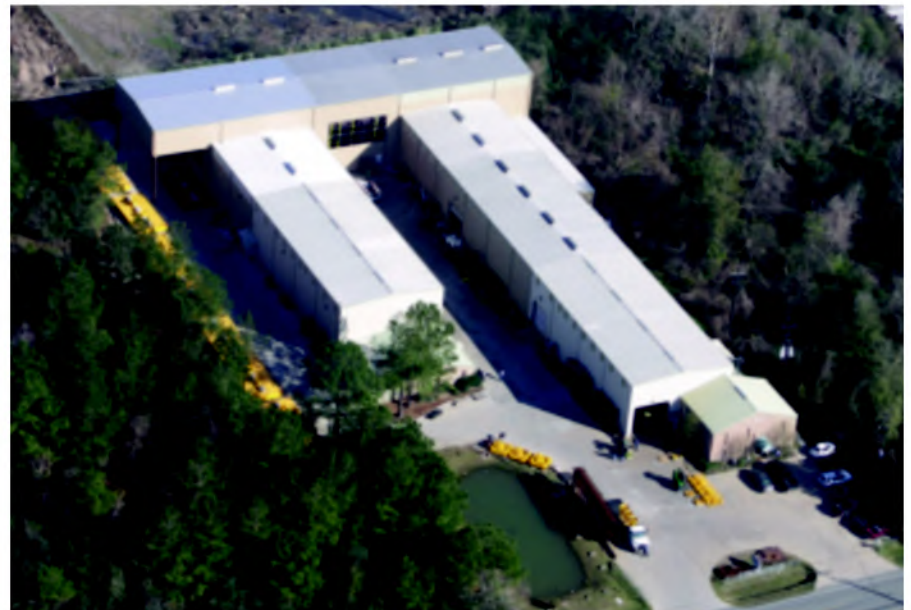
An aerial view of Duron Systems, Inc., a steel fabricating company that has become the first AWS CWF in the Houston, Tex., area.
