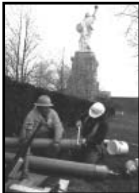
Trim spigot end before attaching pulling eye.
