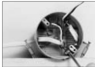
Make Grounding Connection
