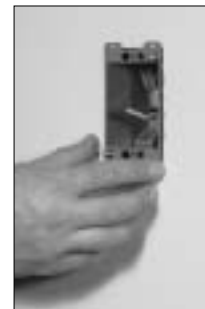
Place Box in Wall
