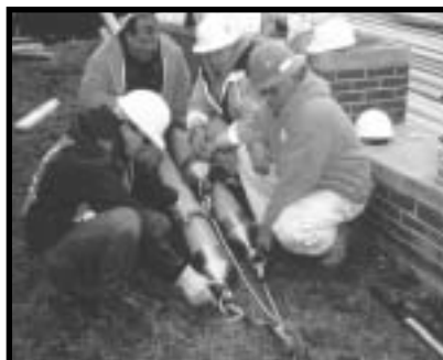
Tighten pulling eye so that it expands against interior of the conduit.
