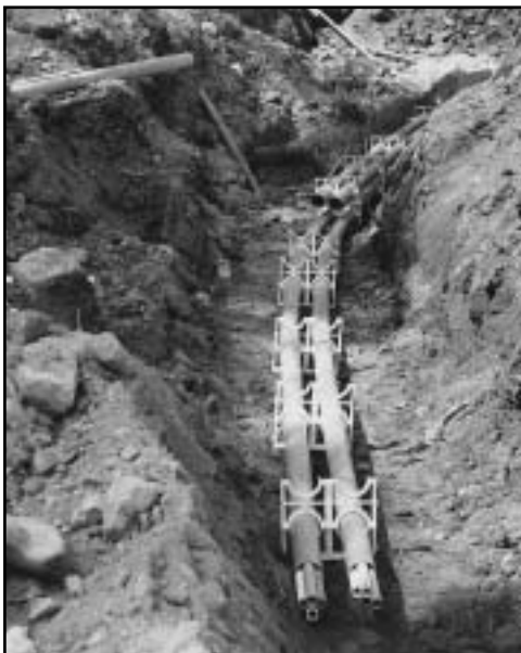
Pulled through existing conduits
