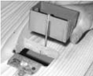
Install clip over subfloor.
