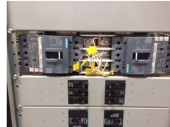
3VA52 3VA61/2 – 150A/250A (DG/FG/FD successor) in P4, P5, SWBD
