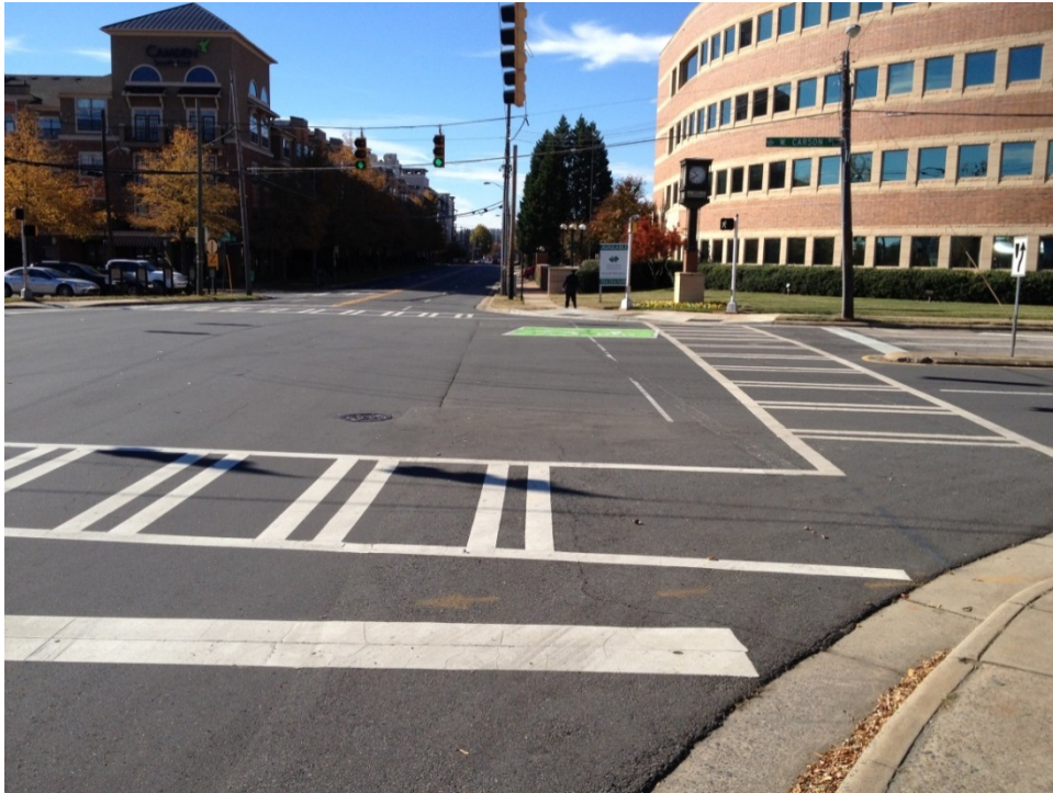
Figure 3: Two-stage left turn box from cyclist's view to turn left onto side street.
