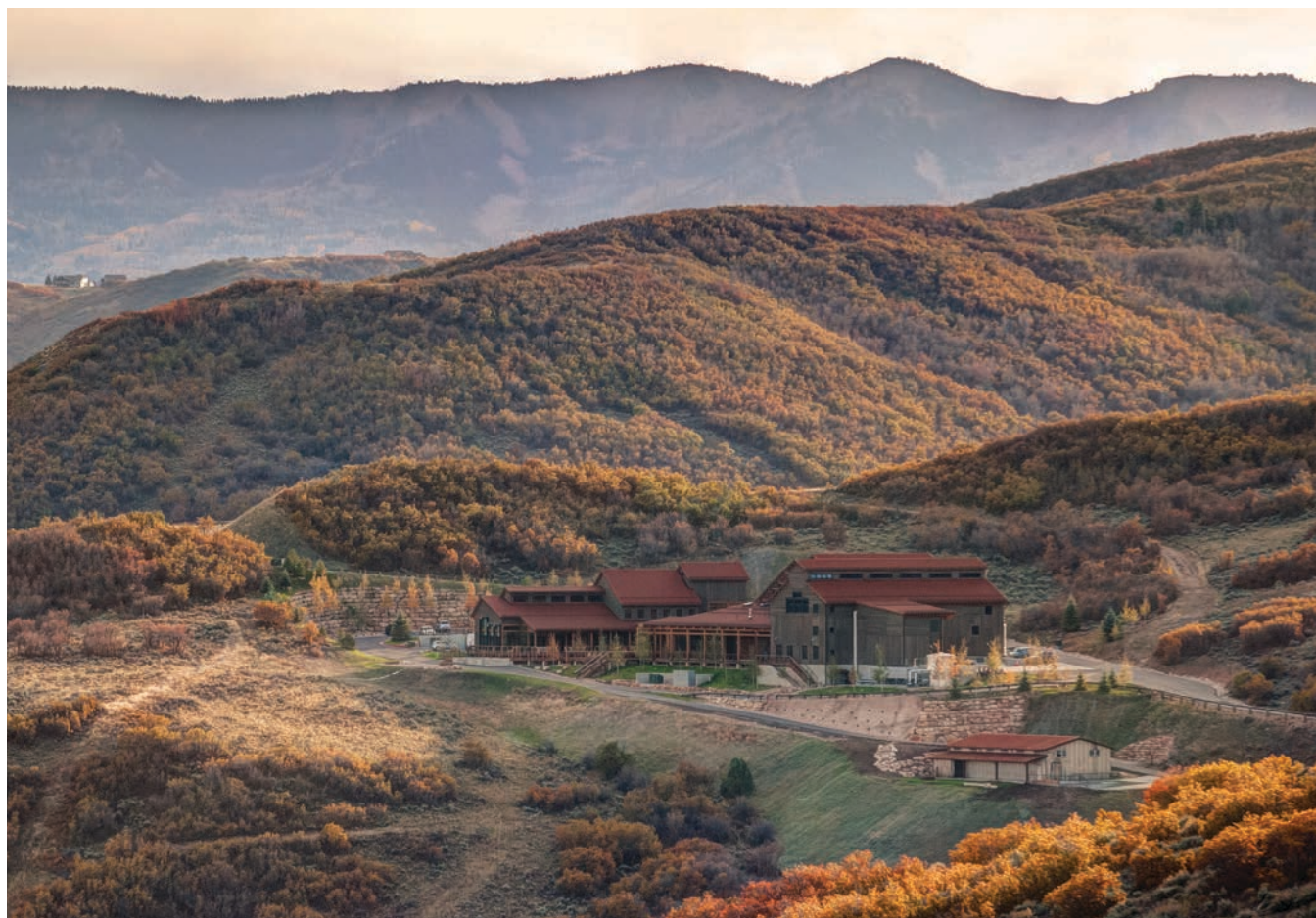
Perched on a hillside in Park City, Utah, High West Distillery's new 30,000-square-foot facility was designed to look like an old mining building.
