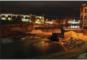
Jackson Mills Dam
