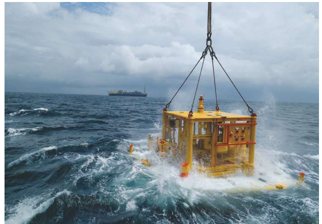
A flowline end termination attached to an XT tree is deployed offshore. (Source: Ulric Ibanez)
