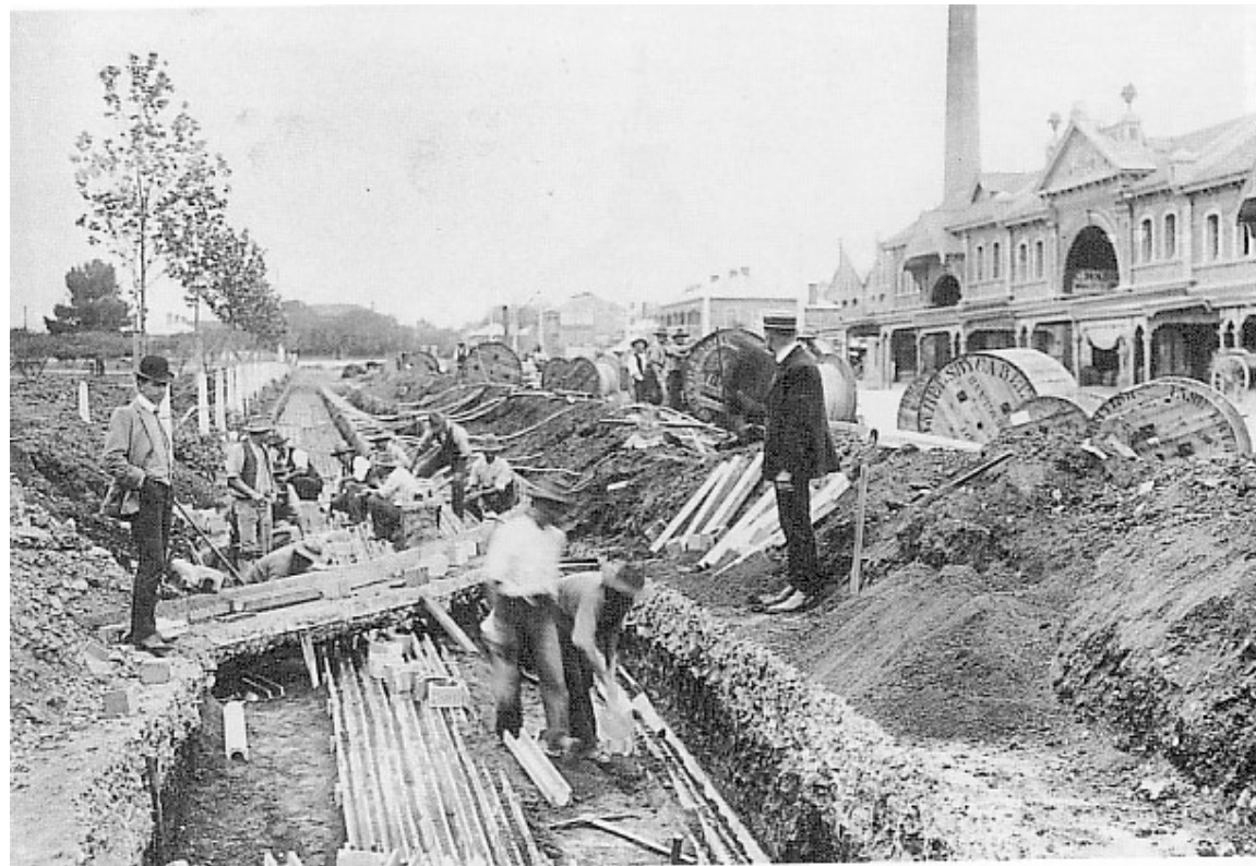
Figure: Laying electricity cables in East Terrace in 1907-08. Note the white painted post and wire fencing and the young Plane Trees ( Platanus orientalis ) to the left. Source: ACC Archives.
