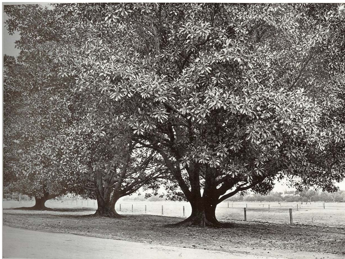
Figure Photograph of three Moreton Bay Figs ( Ficus macrophylla ) specimens on the northern side of War Memorial Drive in 1928 looking northwards. These three trees exist today very close to the Montefiore Road intersection. Note the open paddock behind that is now landscaped as part of the Golf Course. Source: ACC Archive.
