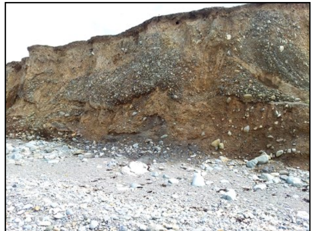
Figure 2. Gravel beds massively broken up.
