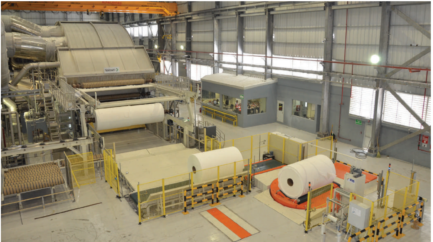
Responding to customer demand: the new TM that started-up in 2015 boosted the company's Mexican tissue production by 60,000tpy
