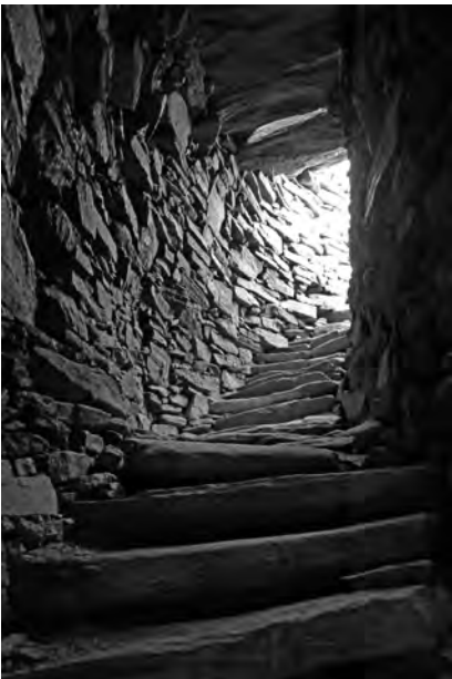
Under: corbelled dome in the “guarded cell” in the entrance wall. Corridors as corbelled arches.
