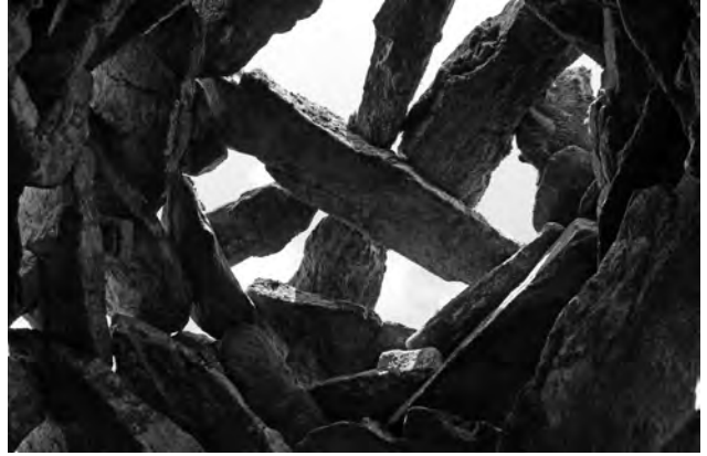
Makeshift roof with large stone beams.
