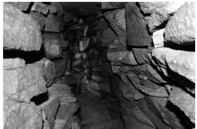
Under: corbelled dome in the “guarded cell” in the entrance wall. Corridors as corbelled arches.
