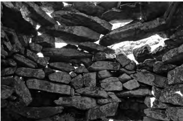
Recessed niches in the wall at ground level, where the wall is especially thick.
