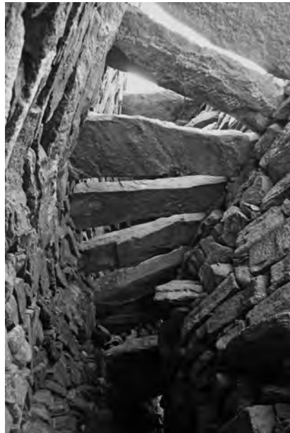
Under: corbelled dome in the “guarded cell” in the entrance wall. Corridors as corbelled arches.
