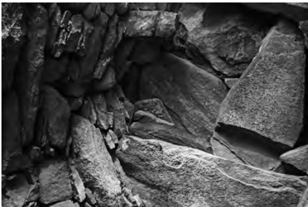
Under: corbelled dome in the “guarded cell” in the entrance wall. Corridors as corbelled arches.
