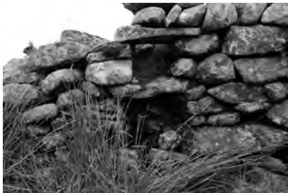
Portable covering stones on the roof. In the background are further ruins.
