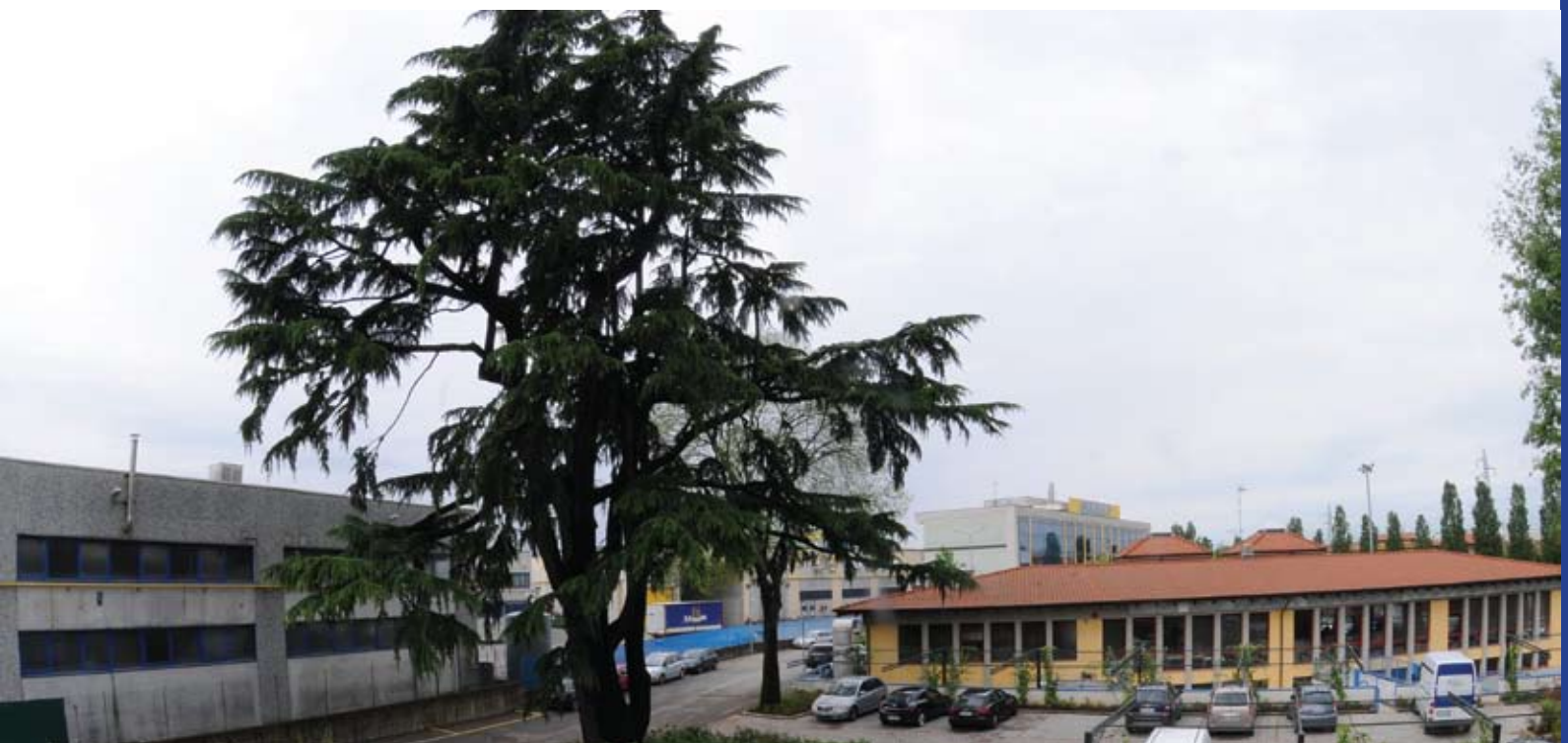
Sabaf headquarters in Italy
