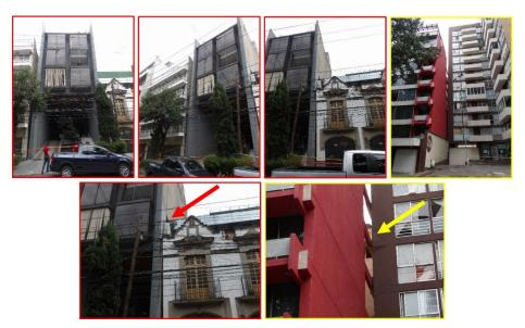
**Figure 16**: Damage induced by pounding between closely spaced buildings due to the September 19, 2017 earthquake (from Lekkas et al. 2017).
