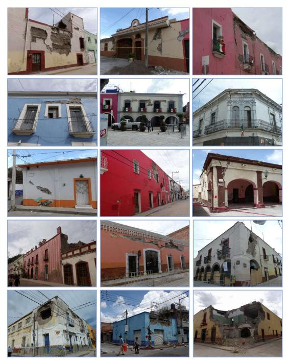
Figure 18: Non-structural and structural damage induced by the second earthquake on September 19, 2017 to the adobe and masonry buildings in Puebla and Morelos states (from Lekkas et al. 2017).
