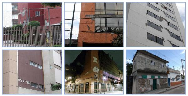
**Figure 11**: Non-structural damage to R/C and mixed type buildings in the affected area due to the September 19, 2017 M 7.1 Puebla-Morelos earthquake. Cracks in the infill walls and detachment of pieces of plaster from the infill walls.
