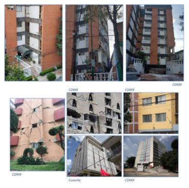
Figure 10: Non-structural damage in RC buildings in Mexico City (Ciudad de México: CDMX) and Cuautla (Morelos State) (From Lekkas et al., 2017).
