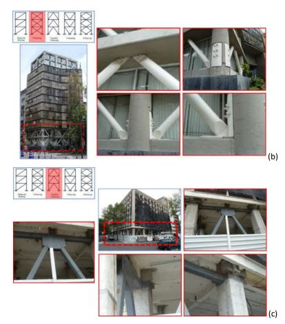
Figure 7: Reinforcement of buildings comprising external steel systems in Mexico City after the September 19, 1985 M 8.1 Michoacán earthquake. There are various types of bracing frames observed such as (a) diagonal bracing, (b) x-bracing and (c) inverted v-bracing frames.
