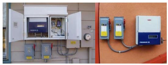
Figure 3: Inverters with their disconnect switches used in PV units (Hellenic Fire Brigade 2015)
