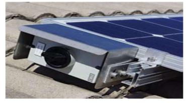
Figure 4: Solar PV system with a rooftop installed DC isolator switch (Chiaramonte et al 2016)
