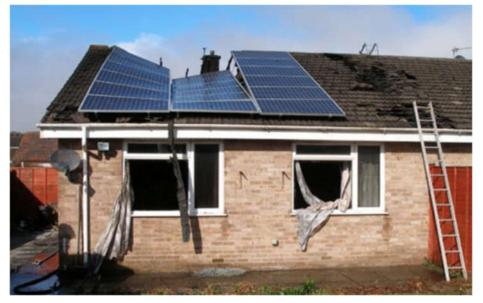
Figure 9: Roof collapse caused by a solar PV system fire (Shipp et al.2013)
