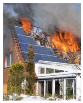
Figure 6. Rooftop PV fire in Scwerinsdorf, Germany in February 2010 (Laukamp et al 2012)
