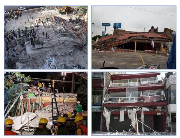
**Figure 14**: Very heavy structural damage (total collapse) of buildings in the Greater Mexico City area induced by the second earthquake in September 2018.
