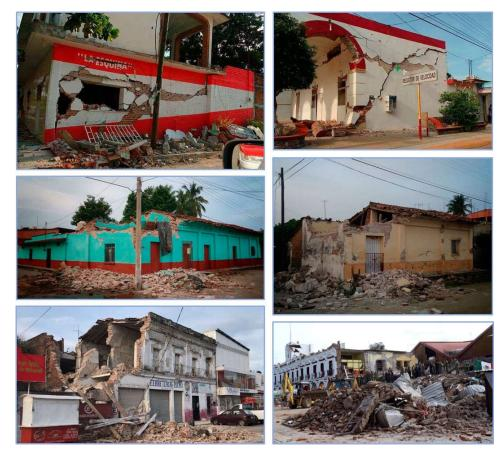
Figure 17: Non-structural and structural damage induced by the first earthquake on September 7, 2017 to the adobe and masonry buildings in Oaxaca and Chiapas states (from Lekkas et al. 2017).
