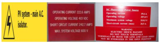
Figure 10. Typical examples of PV sign postings on buildings (Hellenic Fire Brigade 2015)
