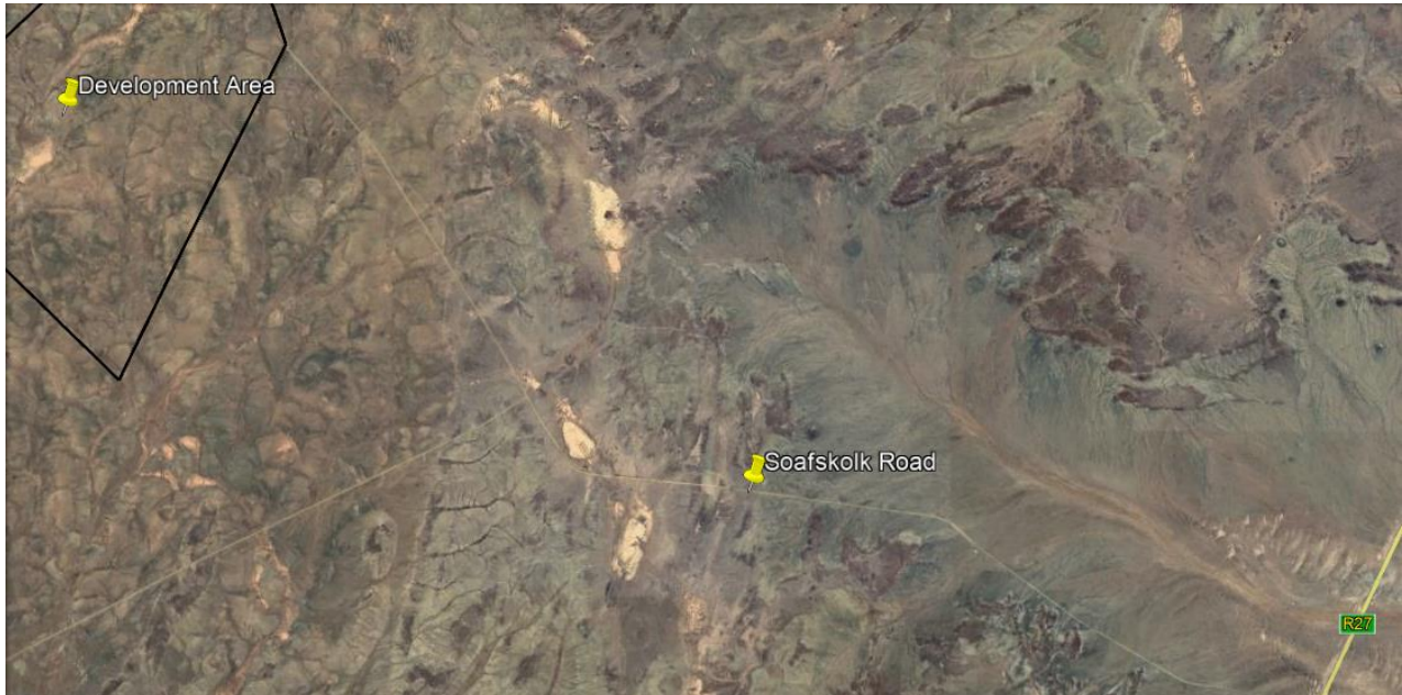
Figure 5.4: Existing road infrastructure within the vicinity of the development area for Kotulo Tsatsi Energy PV3. This infrastructure will primarily be used to gain access to the development area.
