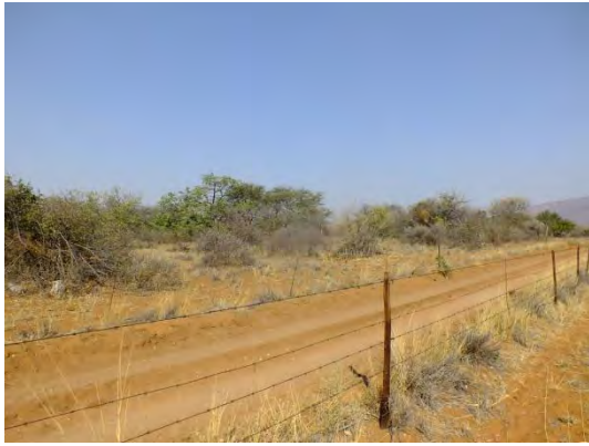
Figure 5-50: Unsurfaced sandy roads typical of the area
