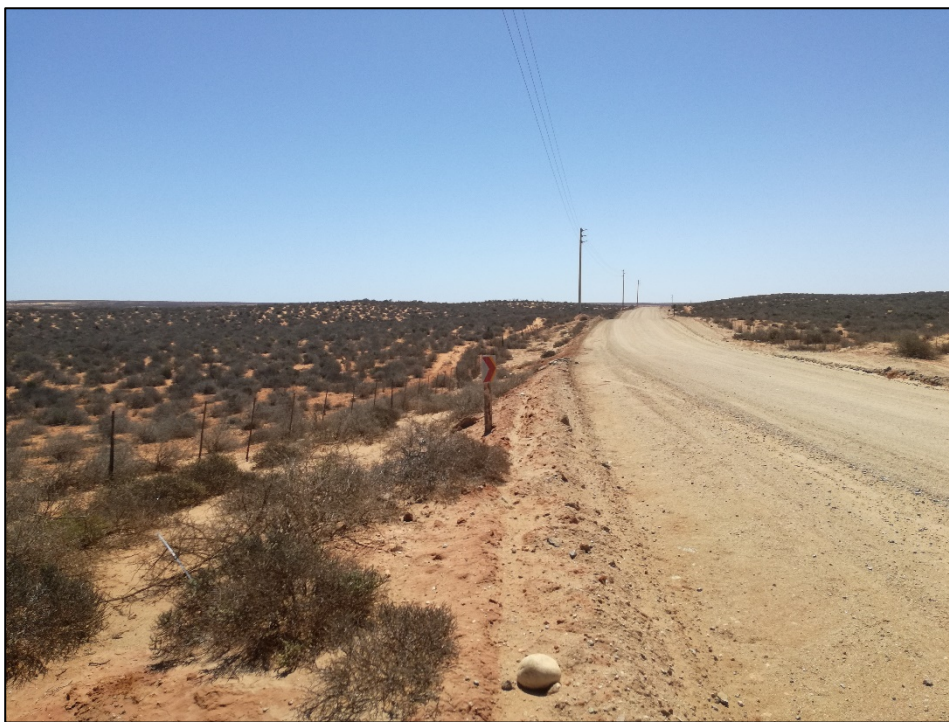
Figure B.16: View of a 66 kV power line along the Komaggas-Kleinsee link road
