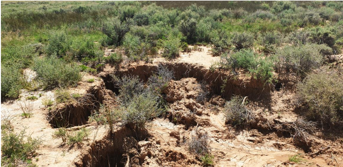
Figure 13: Erosion is occurring in multiple areas along the existing power line servitude, the existing servitudes that are to be utilised must be upgraded with effective erosion control measures to prevent further degradation of habitat.
