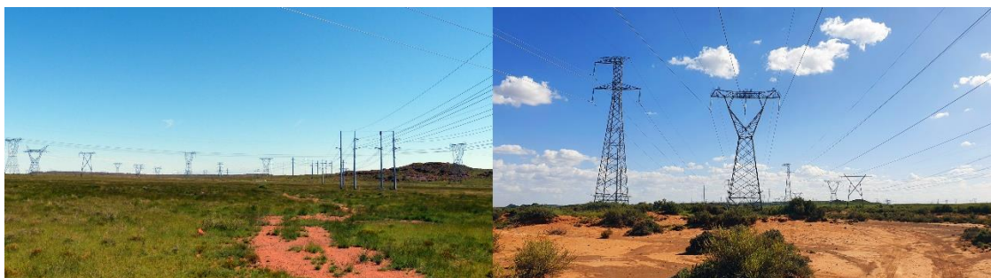
Figure 2: Several existing power lines traverse the area (with associated disturbed areas such as access track and cleared servitudes already existing below the lines). The proposed power line route considered in this proposal follows existing power lines for the majority of its route.
