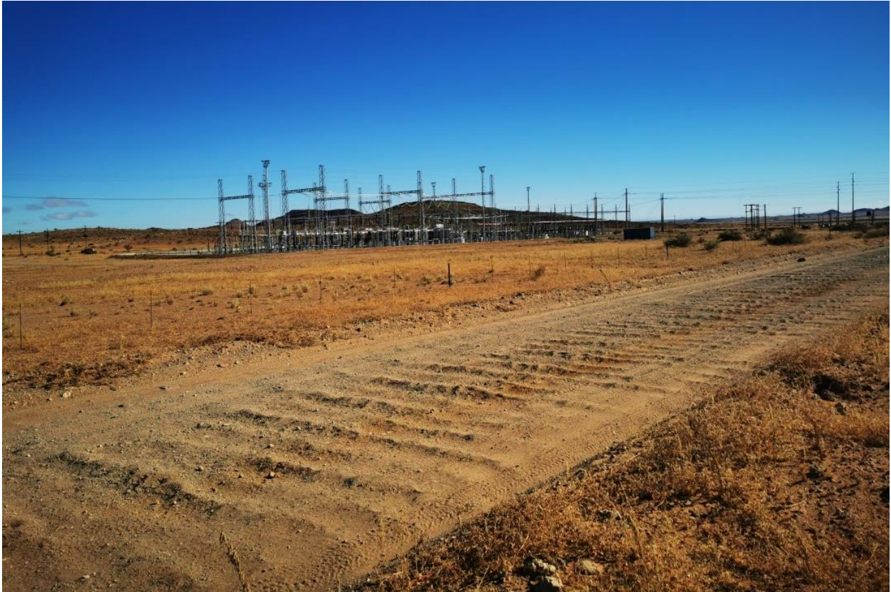
Figure 23 Typical transformed areas (Eskom substation and gravel road towards Onseepkans).
