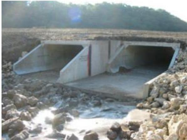
*Figure 6.30: Example of box-culverts that don't allow for corridor continuity.*
