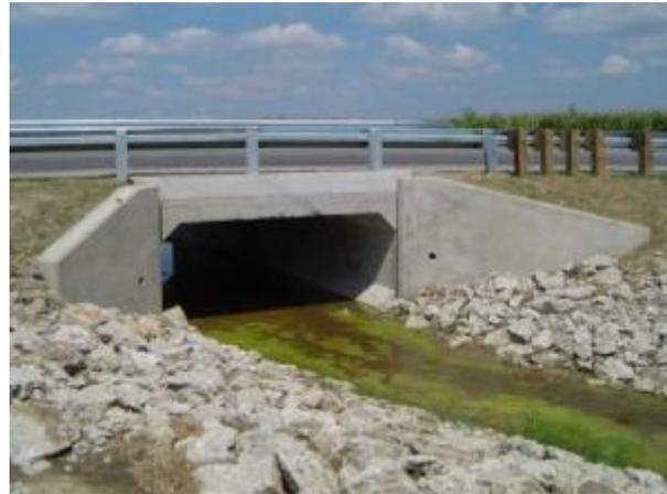
*Figure 6.31: Example of box-culverts that don't allow for corridor continuity.*
