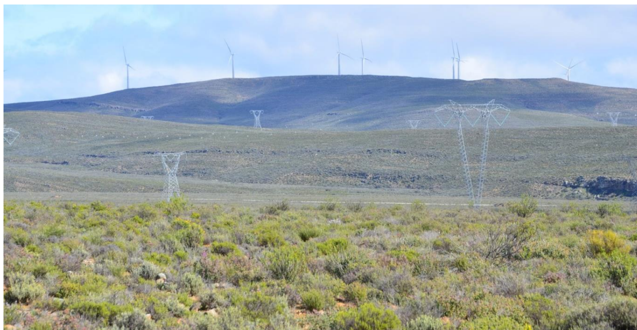
Figure 5-3 Photographs illustrating existing infrastructure within the area.
