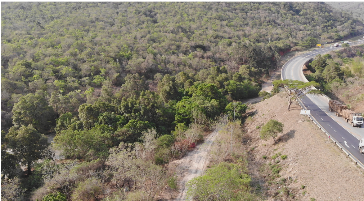
Photo 2: Example of the natural closed woodland/ forest (aquatic) present (Remote Oblique Observation Site 2, Direction North)
