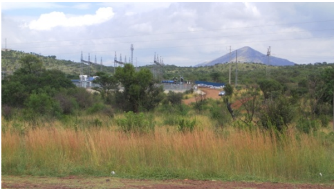
Figure 8: View of natural vegetation and impacts at the Lebowakgomo substation.
