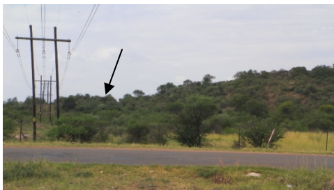
Figure 28: The koppie just to the north of the new Dithabaneng substation with the point where the line will cross indicated by the arrow.
