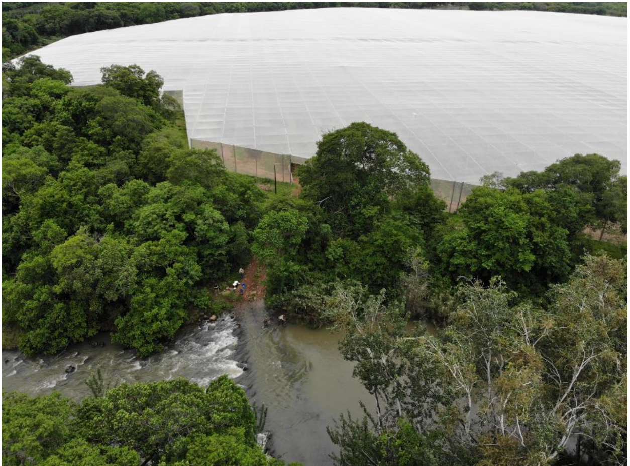
Photo 9: River crossing two showing the low water crossing (rocky drift) and associated infrastructure
