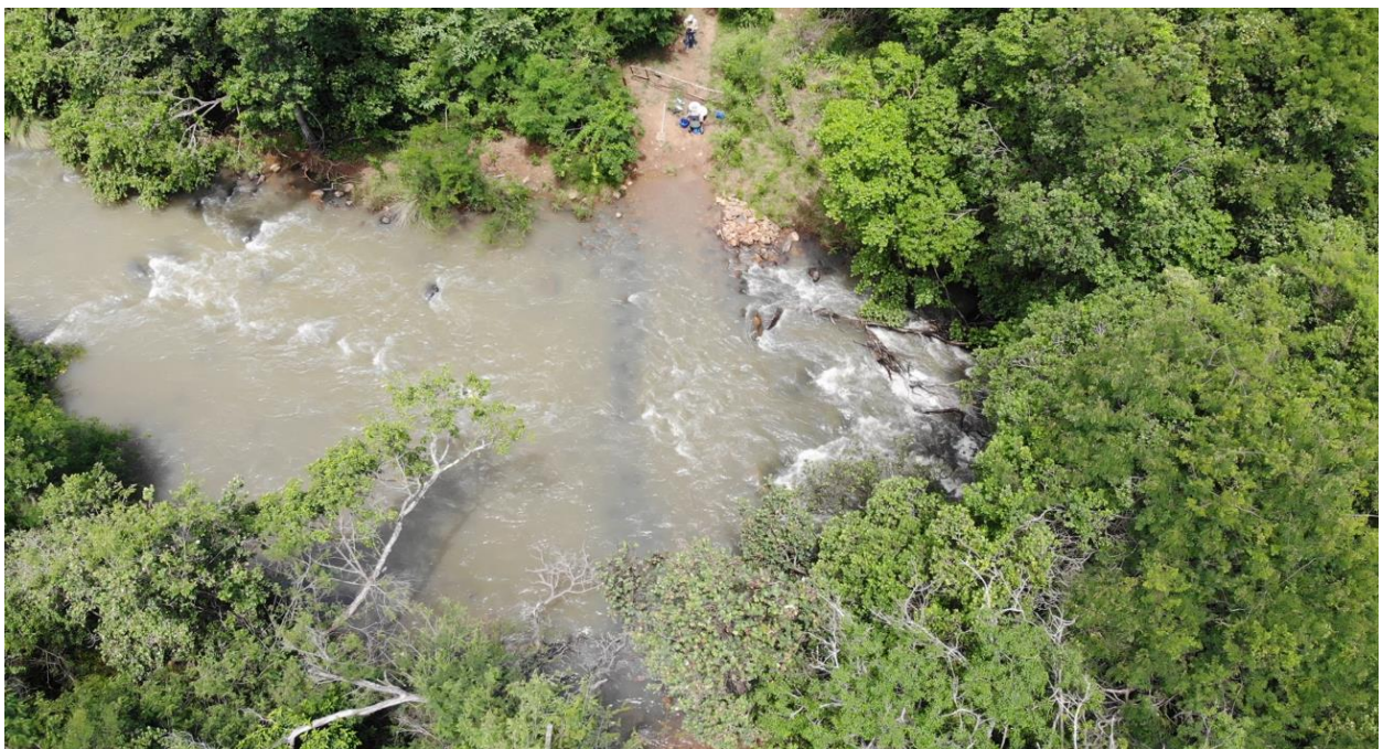
Photo 8: River crossing one clearly showing the low water crossing (rocky drift)
