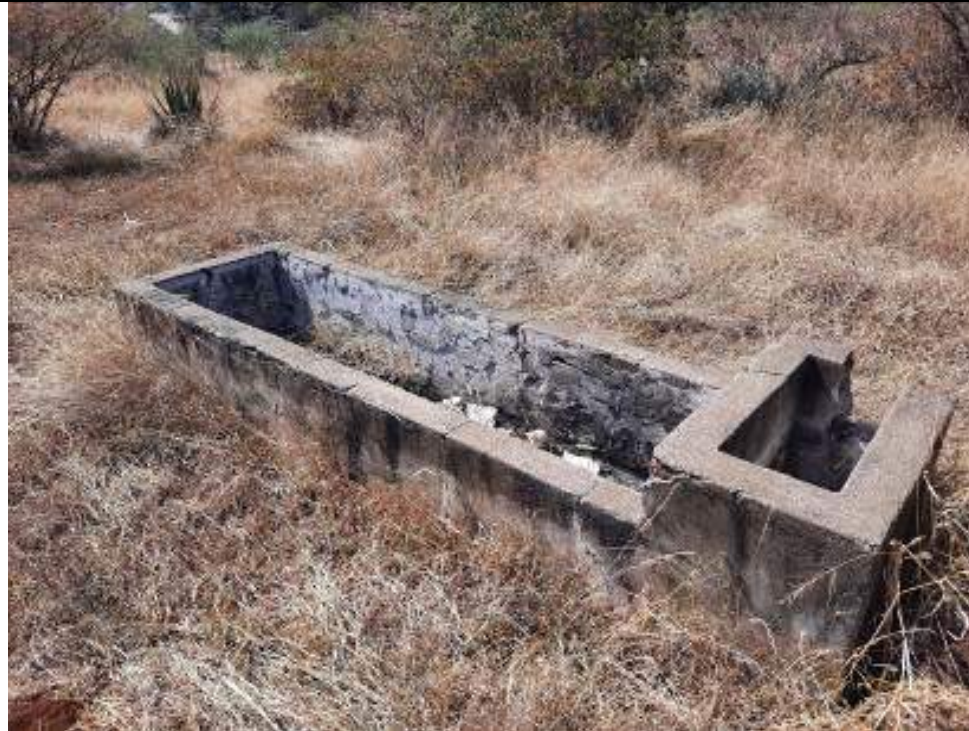
Figure 17 - Cement water trough at Site 1-3
