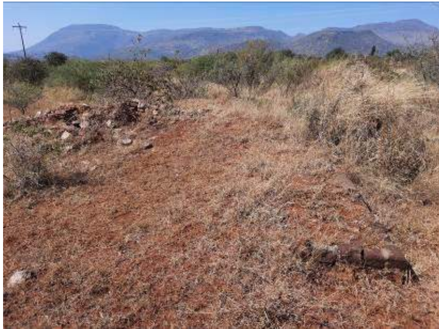
Figure 18 – A series of broken-down structure and foundations.
