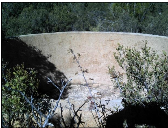
Reservoir to be used as pool for Overnight Camp 1 Photo 5
