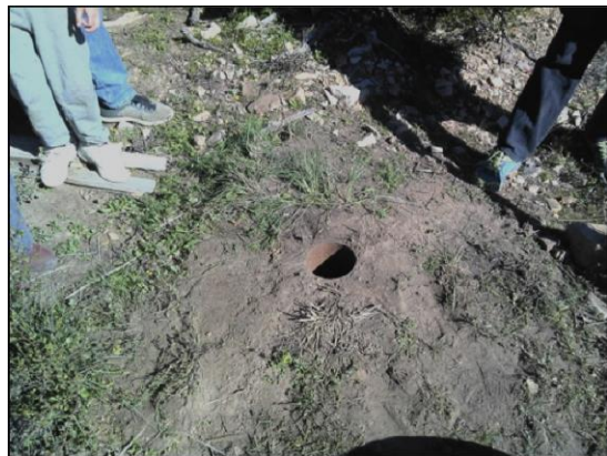
Borehole for Overnight Camp 1 Photo 4
