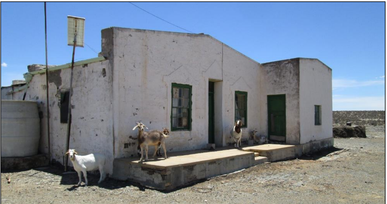
Figure 19: View of the front of the house at waypoint 014. The original south-facing structure is in the centre and has rustication around the windows and front door. It is likely late 19 th century. The
