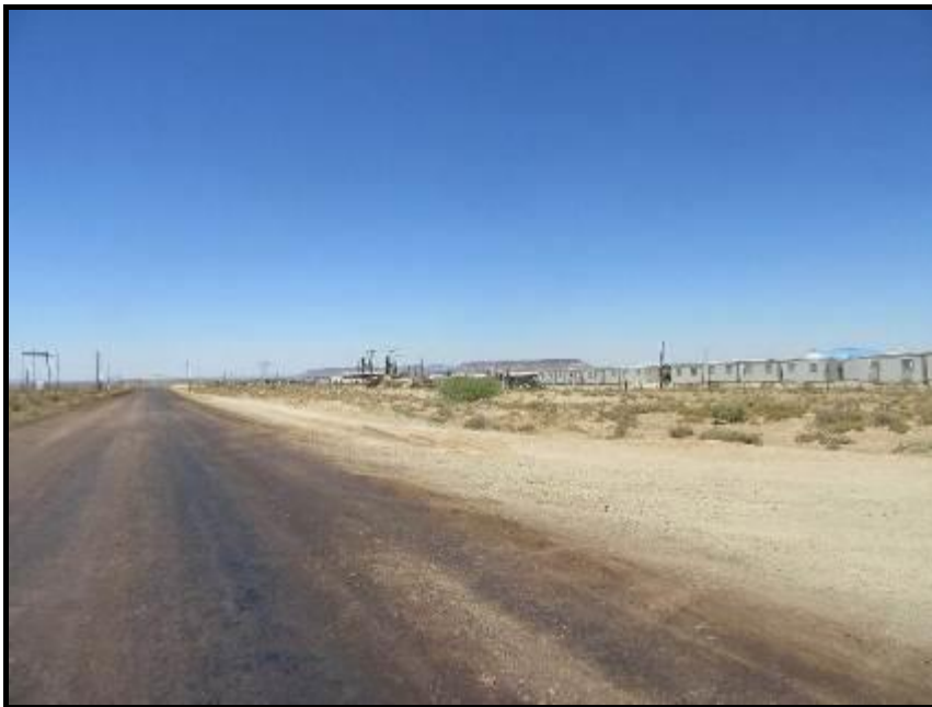
Photograph 1.17: Khobab and Loeriesfontein WEFs construction camp along the Nuwepos Road. Note dust suppressant which has been applied to the road
