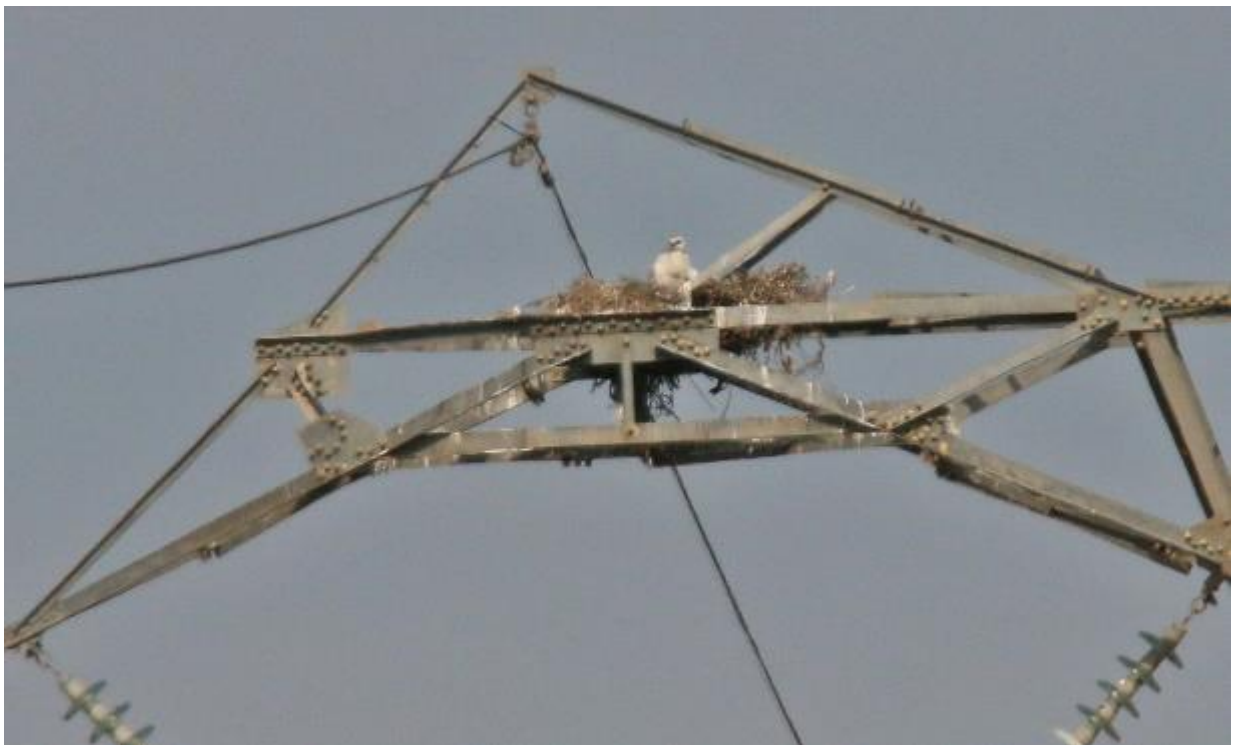
Figure 4: An active Martial Eagle nest on the Aries – Helios 400kV transmission line.
