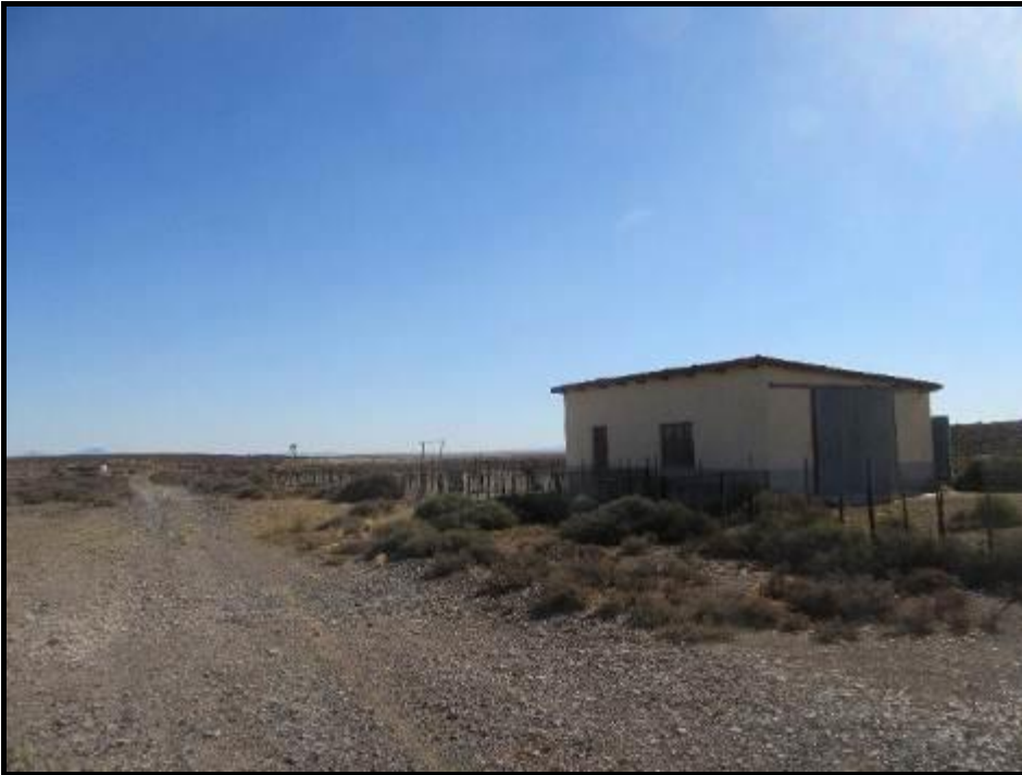
Photograph 1.15: Shed, cement dam and windmill on Harderant
