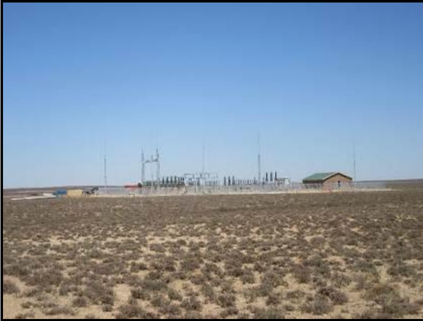
Photograph 1.18: Khobab WEF project substation adjacent to Nuwepos road, currently under construction
