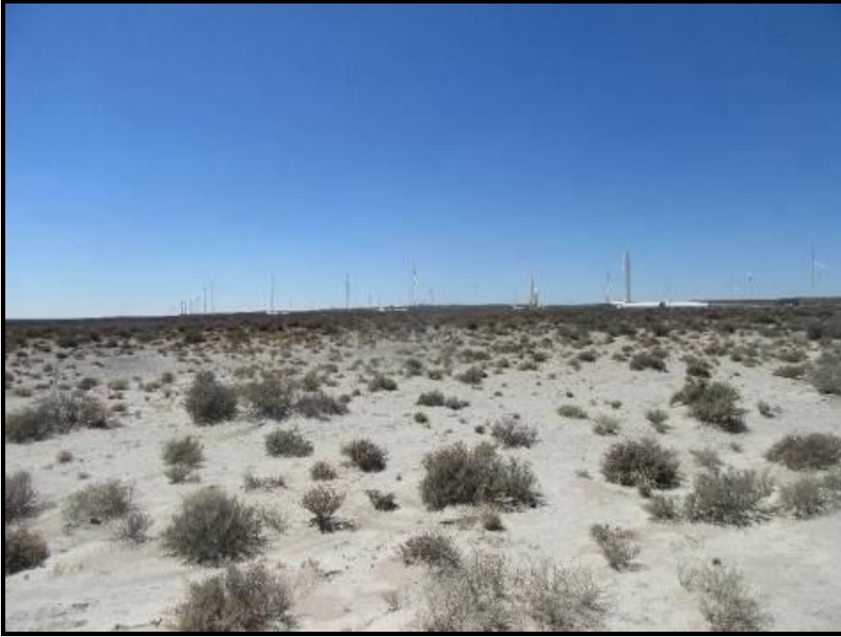
Photograph 1.23: Turbines under construction on Loeriesfontein WEF on Kareedoorpan (Lintvelt) east of the Nuwepos road
