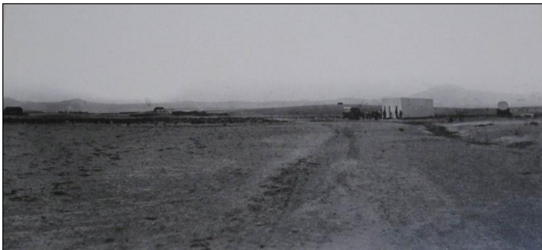
Figure 7: The first building in Loeriesfontein as photographed in 1895 (Source: Fred Turner Museum, Loeriesfontein).
