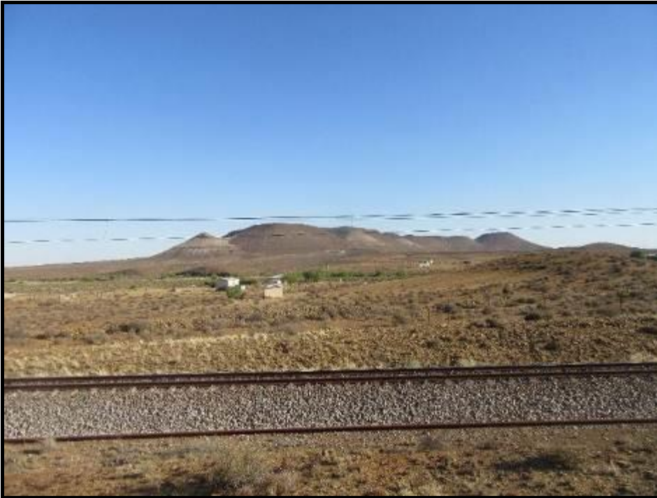
Photograph 1.12: Houses on Klein Rooiberg and Klein Rooiberg-Wes, viewed from across the Sishen-Saldanha railway line
