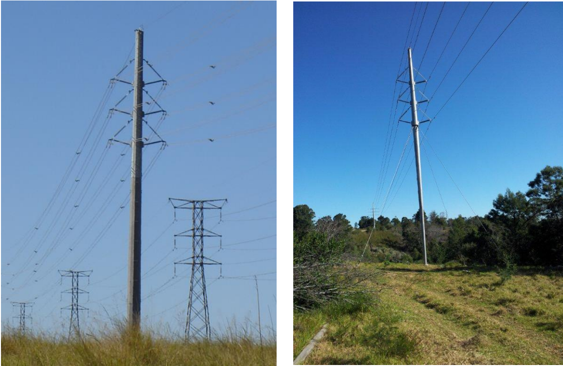
Figure 3: Example of a 132kV double circuit self-supporting monopole (left) and a 132kV double-circuit guyed monopole (right)
