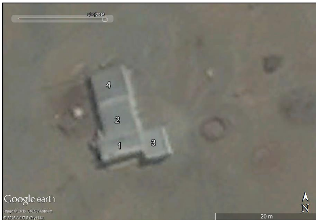
Figure 20: Aerial view of the house at waypoint 014 with the four phases of construction labelled. The small kookskerm is visible as a circle to the east of the house. Source: Google Earth using Bing Maps overlay available at: http://ge-map-overlays.appspot.com/bing-maps/hybrid .
