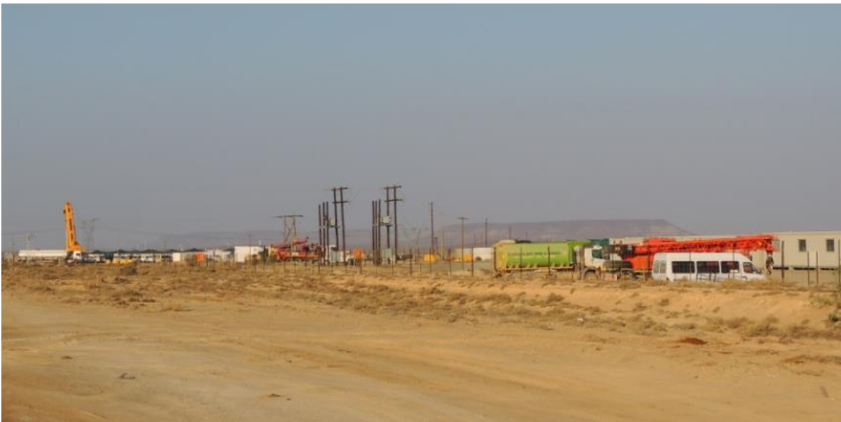
Figure 18: Existing wind farm construction camp adjacent the gravel road.
