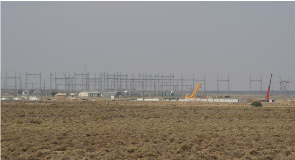
Figure 13: Photograph of the Eskom Helios substation and the Mainstream wind farm construction camp in the foreground.
