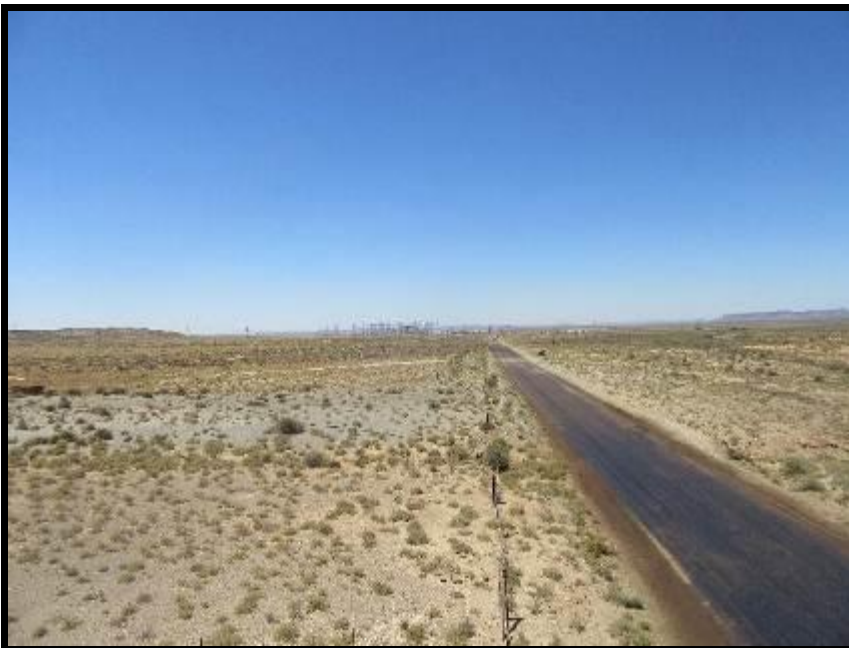
Photograph 1.19: Powerlines entering Helios from both sides of the Nuwepos Road, viewed from the Sishen-Saldanha railway bridge
