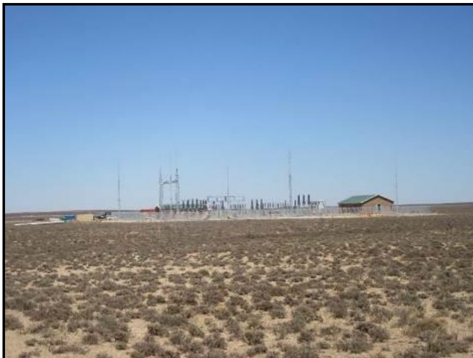
Photograph 1.24: Khobab WEF project substation under construction
