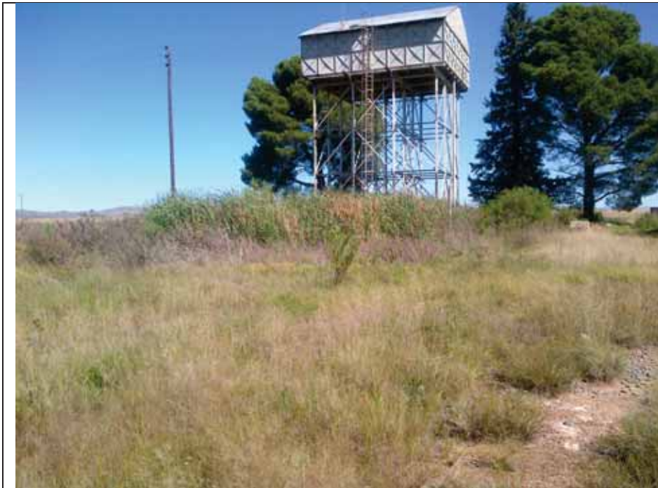
Historical water towers positioned next to the existing railway line at Visrivier area
