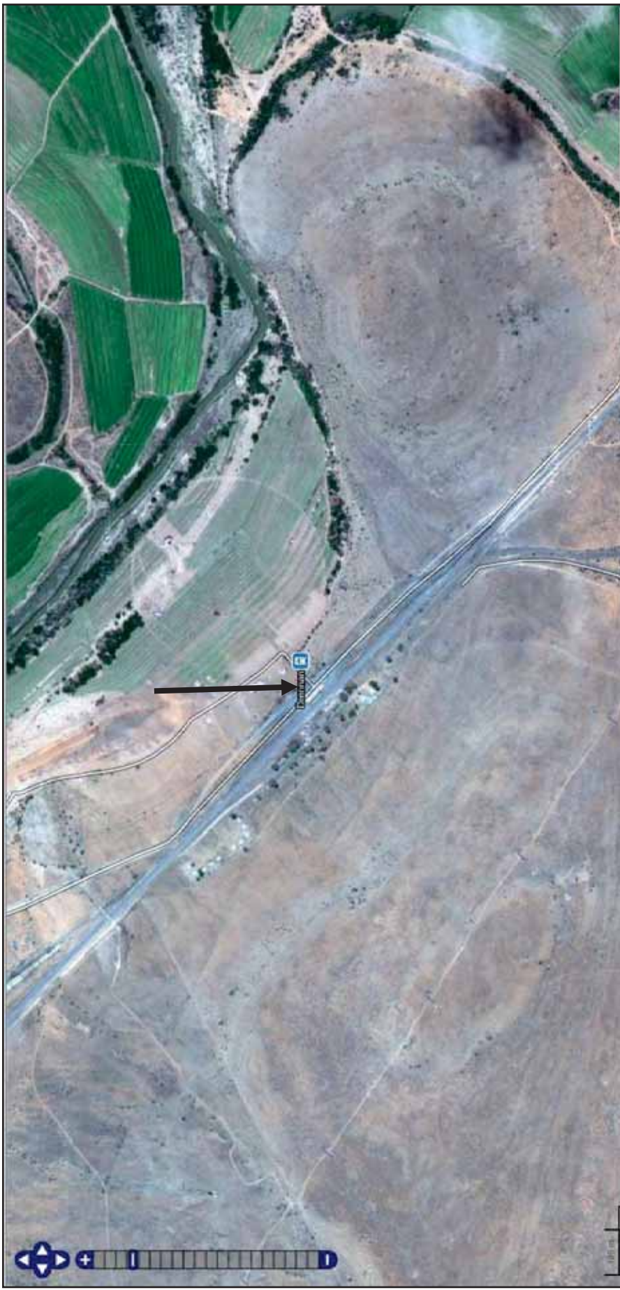
Figure 35: Aerial view of the proposed Drennan loop extension (SAHRIS, 2013)
