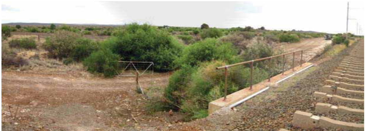
Figure 19: Illustrates an alluvial fan/ wash crossing (map label 22) located approximately 210 m east of the Tsantsabane loop extension. A channel is not clearly defined, but convergent contour lines are present, which indicate that surface flow is concentrate in the area after sufficient rainfall events.
