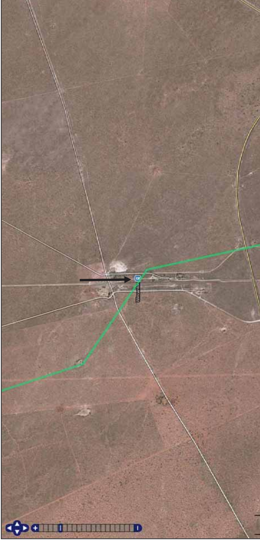
Figure 5: Aerial view of the proposed loop extension at Wincanton Station (SAHRIS, 2013)
