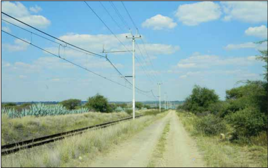
Figure 69: The railway reserve south of Fieldsview Station
