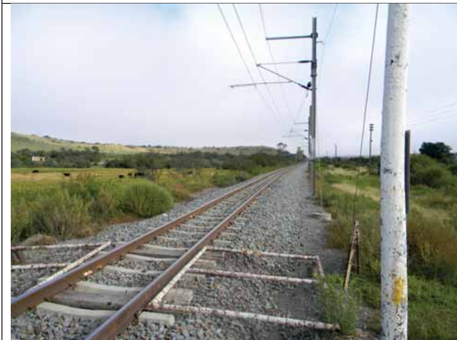
Railway crossings at Kommadagga
