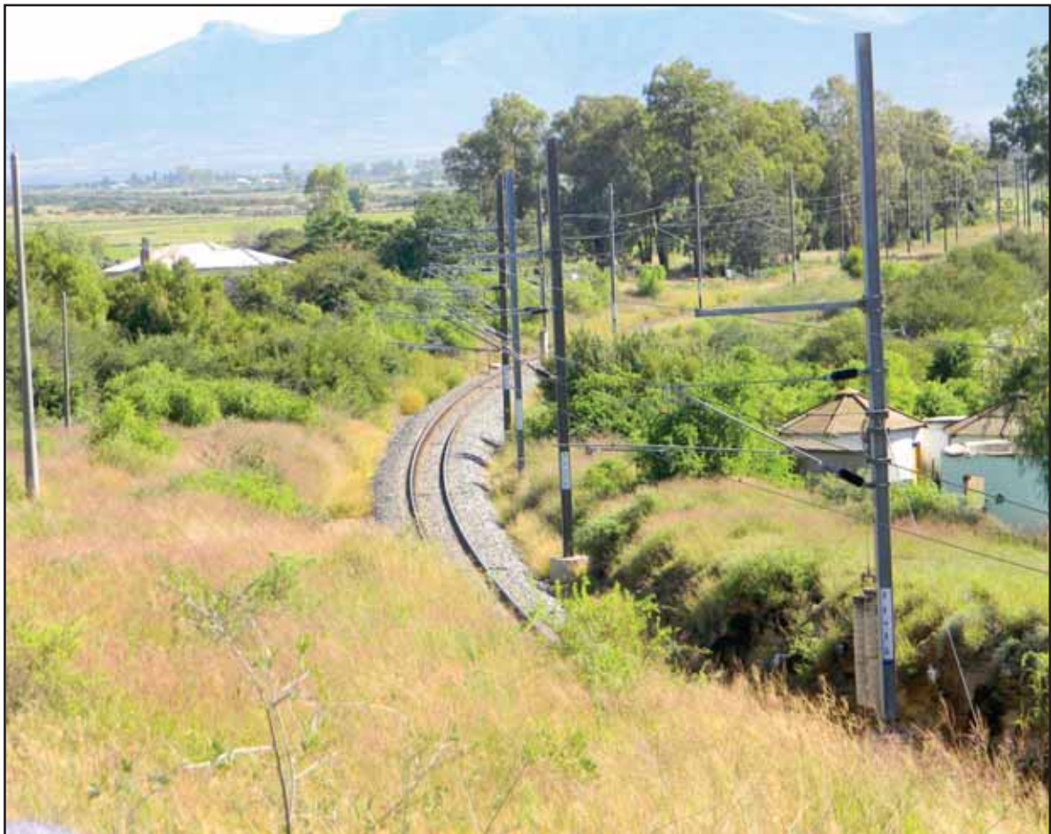
Figure 86: Railway line south of Golden Valley Station. Historical and temporary structures are situated alongside the existing railway line
