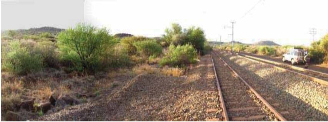
Figure 31: Illustrates a culvert crossing in the northern section of the Glosam loop with no drainage line or watercourse crossing present.
