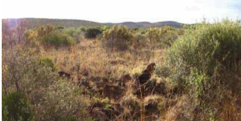
Figure 29: Illustrates a culvert crossing in the southern section of the Glosam loop; a man-made channel has been made to drain sheetwash away through the raised embankment and culvert (top). This creates the impression of a natural channel, but the channel feature disappears a short distance away from the railway line (bottom). No natural drainage line features were identified on aerial photographs or on site.
