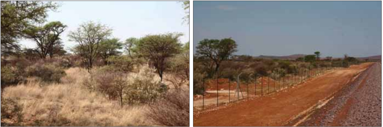
Figure 5. The Sishen site, illustrating the dense nature of the intact vegetation at the site, as well as the extent of cleared ground that has been created by construction activities for the new line at the site, being built by Kumba Iron Ore.
