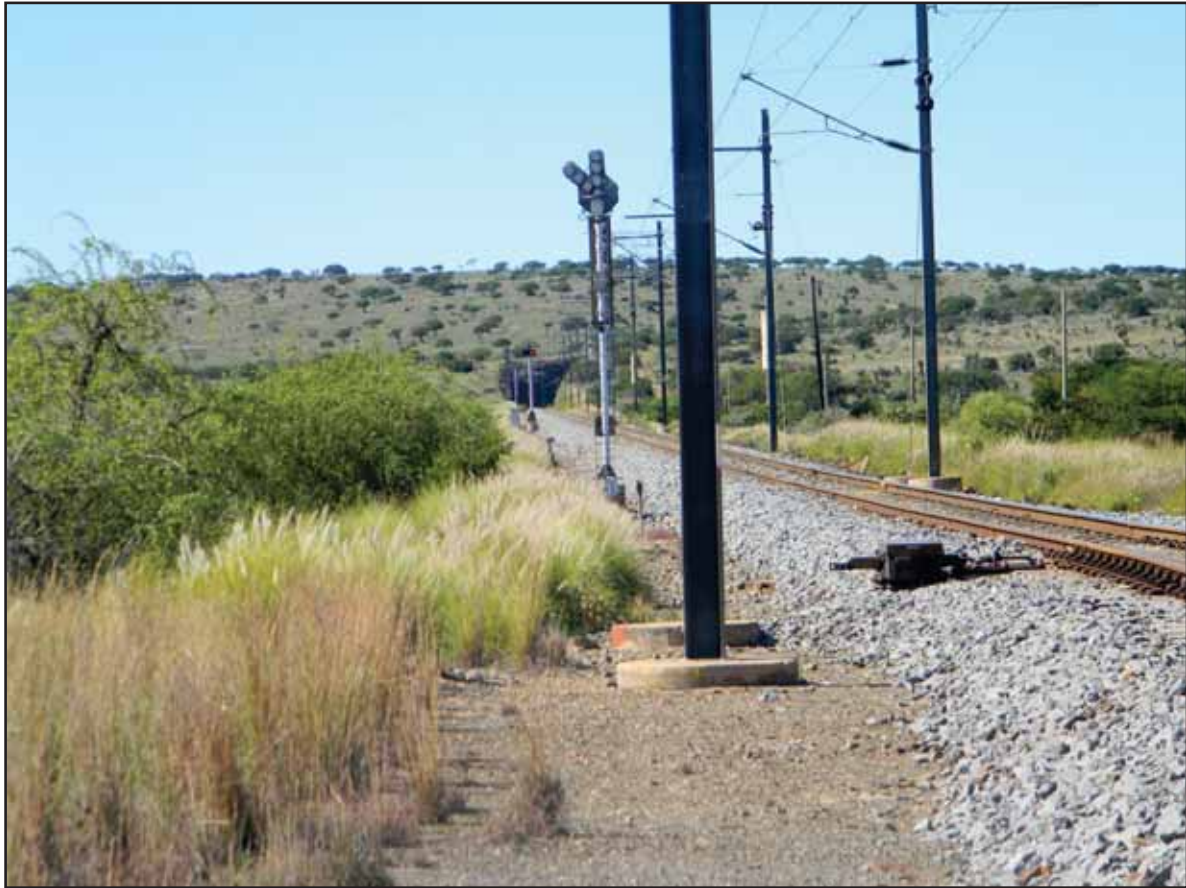
Figure 102: Railway line positioned south of Kommadagga Station
