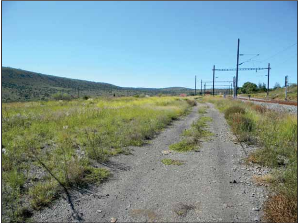
Figure 96: Railway reserve road heading towards Kommadagga Station
