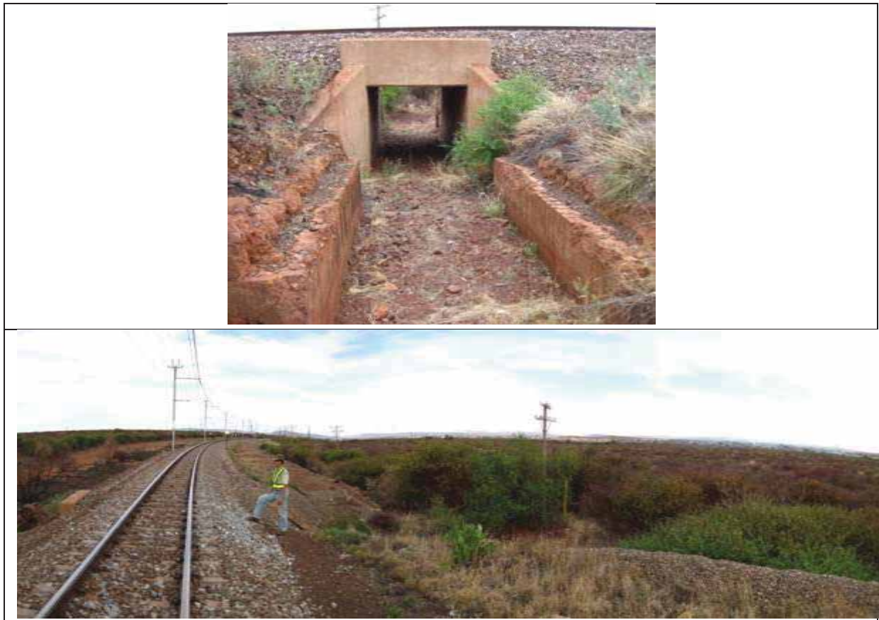
Figure 25: Illustrates an indistinct drainage line crossing in the Postmasburg section (map label 27) with an existing culvert (top and bottom). The drainage line is dominated by Acacia mellifera , while an alien plant species ( Opuntia sp.) is present on the rail embankment (bottom). Ballast material is present within and adjacent to the drainage line (bottom).
