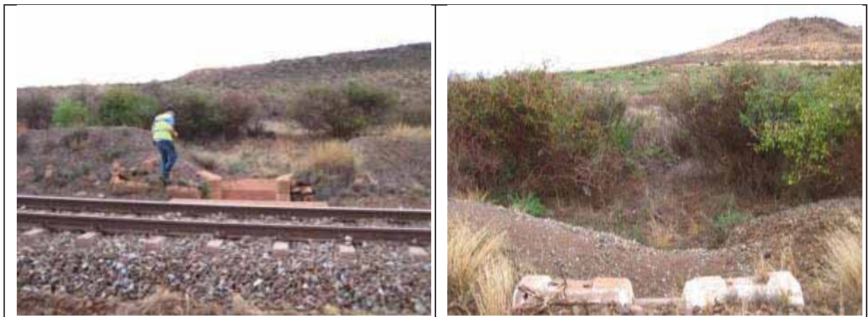
Figure 26: Illustrates an indistinct drainage line that originates approximately 30 m downstream of the Postmasburg loop extension (map label 28), (right). An existing culvert is present along with ballast material downstream of the culvert (left and right). Notice the gap that has been created in an upstream embankment to allow surface flow through the culvert (left).
