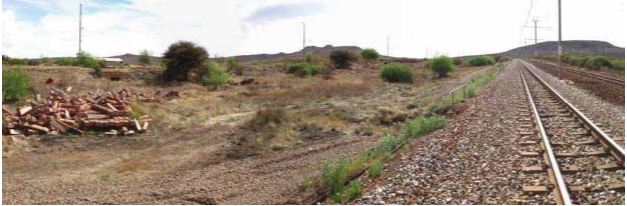
Figure 23: Illustrates an indistinct drainage line crossing in the western section of the Postmasburg section (map label 25), which has been seriously modified through dumping, as well as railway line and dirt road crossings. Exotic plant species, such as Prosopis cf. glandulosa and Melia azedarach are present within the drainage line.
