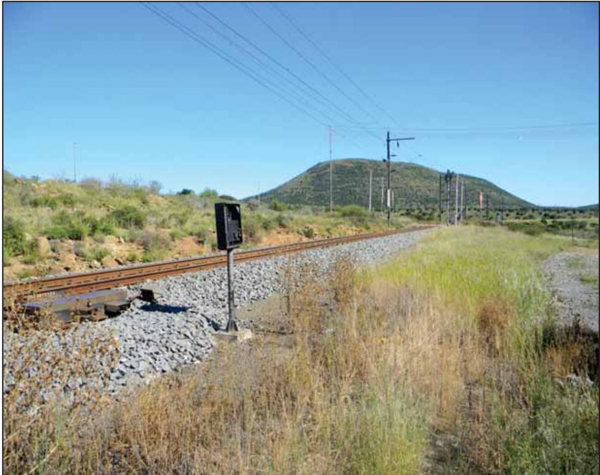
Figure 97: Station and line situated west from the existing railway line at Kommadagga Station
