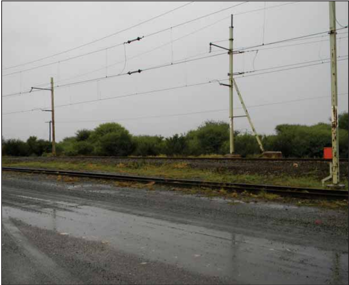
Figure 50: Railway reserve at Ulco Station
