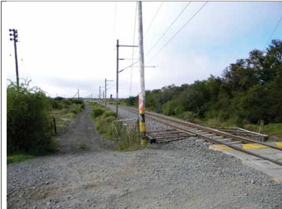
Railway crossings at Kommadagga
