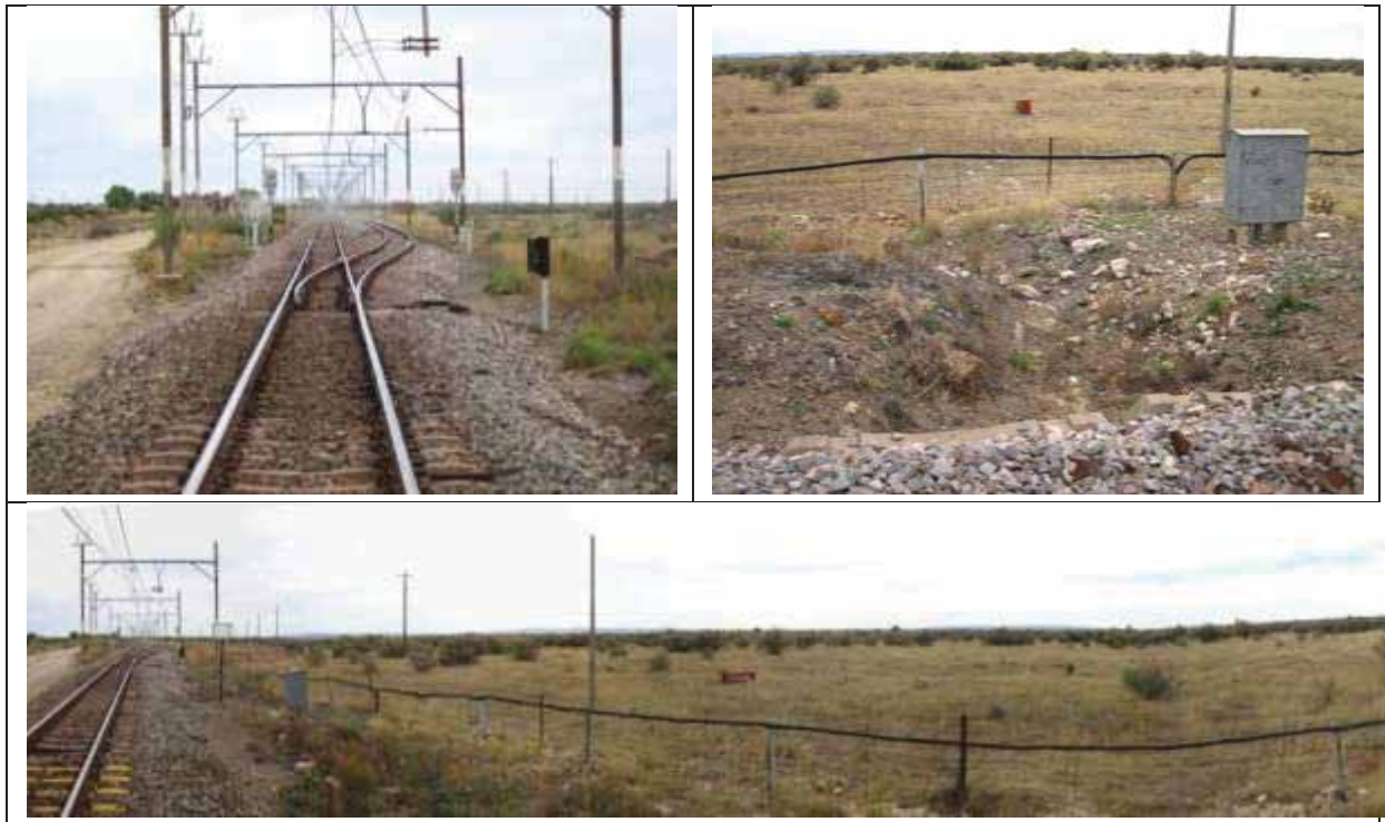
Figure 16: Illustrates the existing Trewil section, which will be extended in an easterly direction for a distance of approximately 1.2 km (top left). A culvert is located \pm 90 m from the start of the proposed new loop extension (top right) and is located in an arid depression wetland (map label 19) that will be crossed by the new loop (bottom). The dry pan does not contain distinct wetland features, apart from a marginally developed terrain unit indicator.
