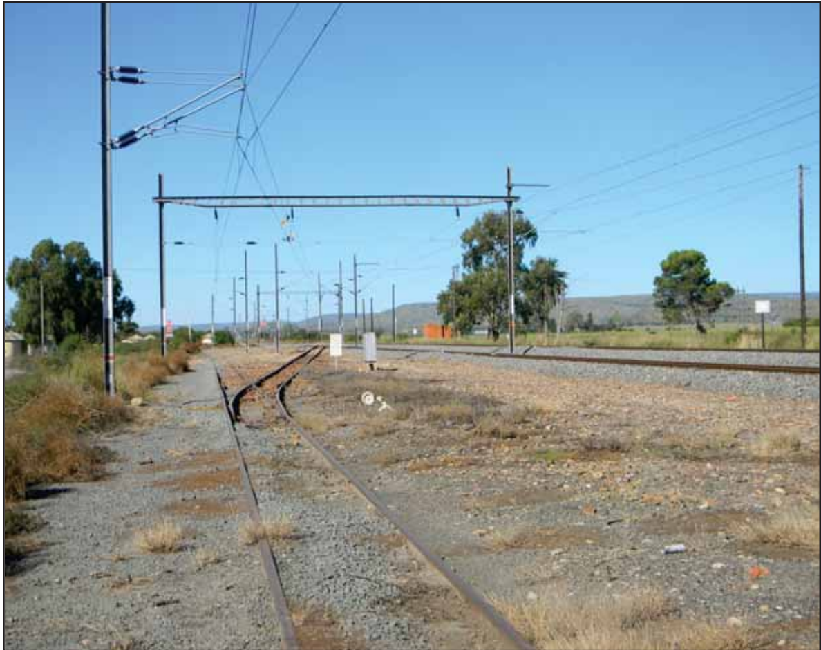
Figure 83: Railway infrastructure at Golden Valley Station
