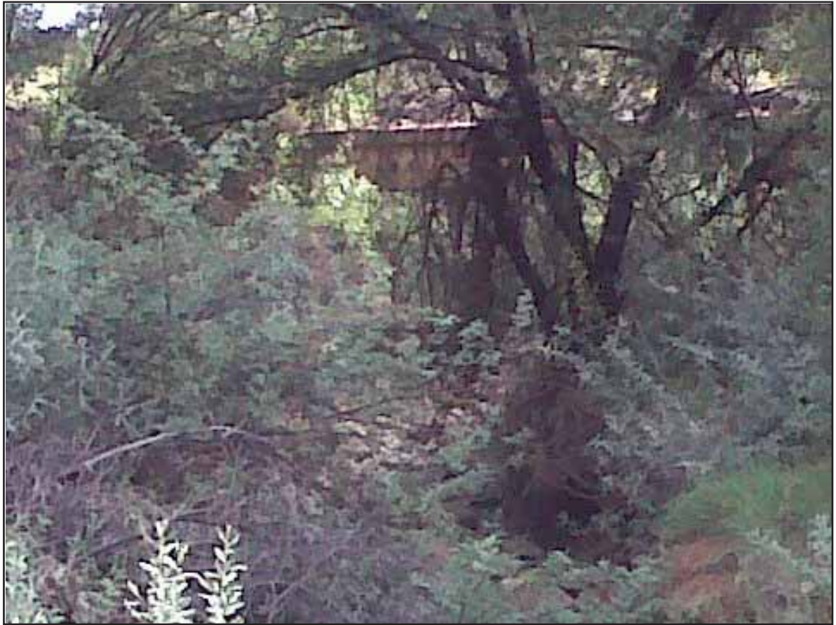
Figure 60: Historical bridge positioned seven metres west of the existing railway line at Gong Gong Station
