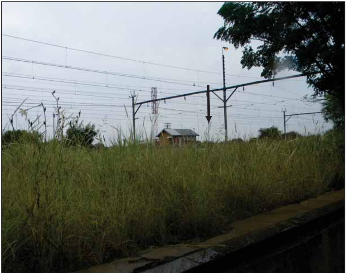
Figure 51: Railway buildings at Ulco Station
