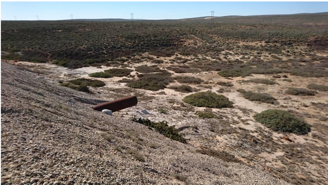
Figure 6 Photos of the main haul road situated 3 km upstream of the mouth within the restricted mining concession area of the WCR. This road prevents the river from reaching the floodplain. Photo A faces upstream and photo B shows how the intake pipe is elevated at least 1 m above the riverbed. Photos were taken on 22 June 2016.
