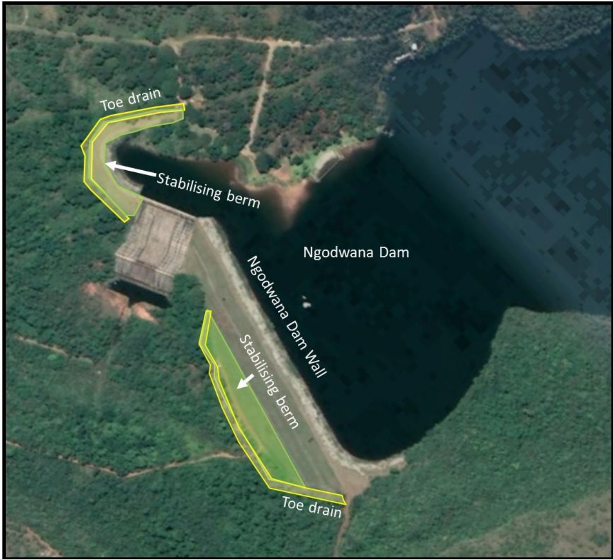
Figure 46: Dam wall berm and toe drain to be stabilised.
