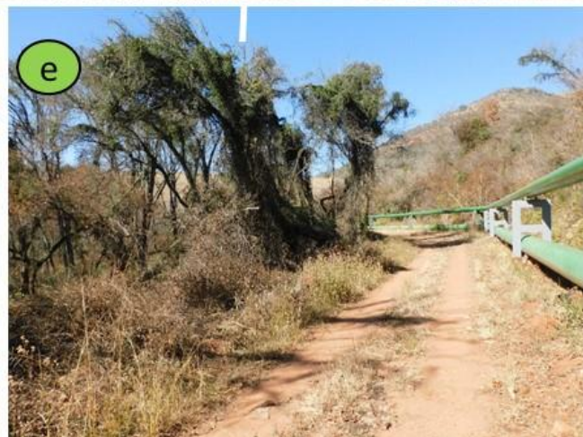
#8 New haul route up the embankment of the dam.
