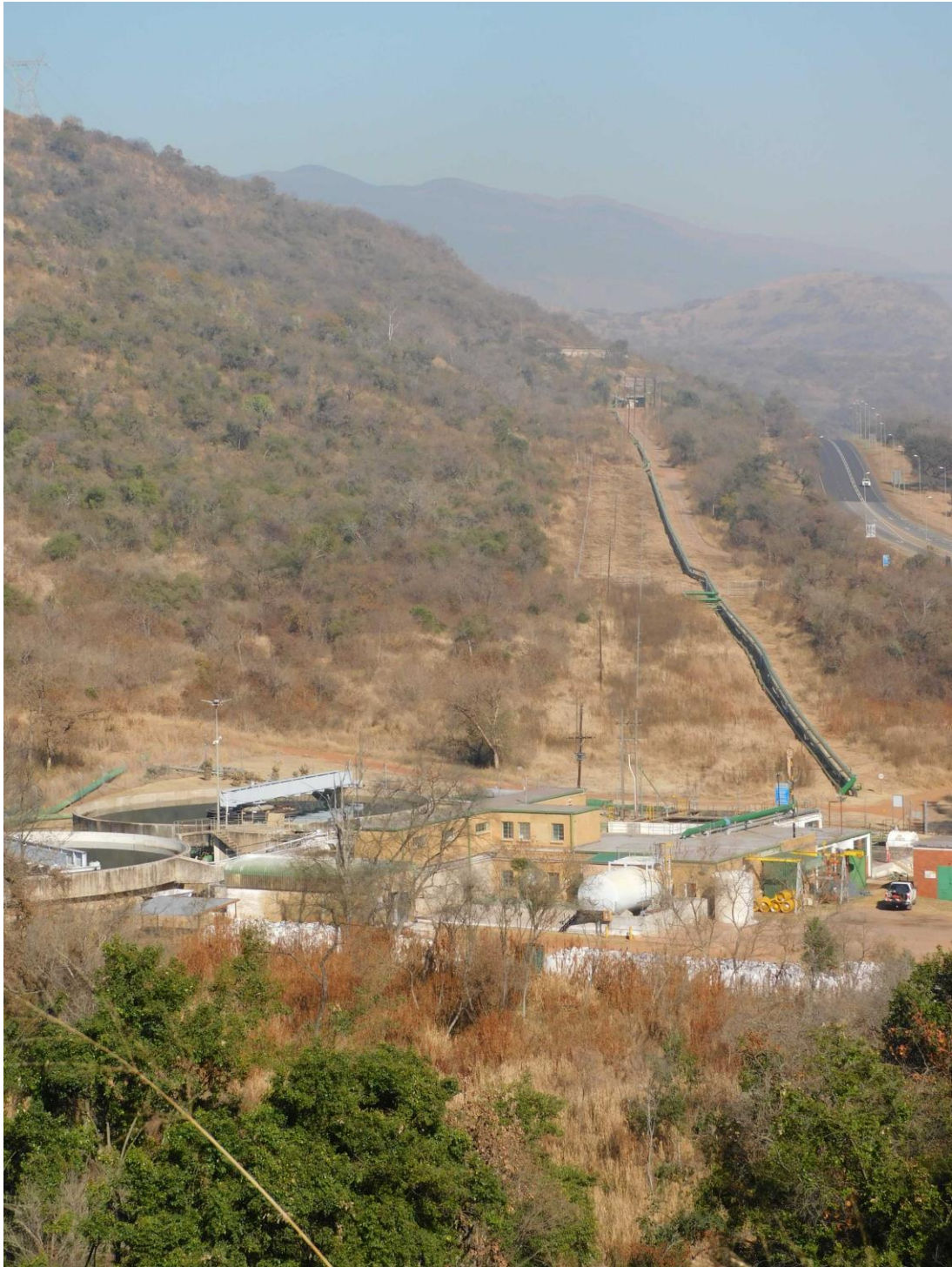
Figure 29 a: The Power Line Servitude.
