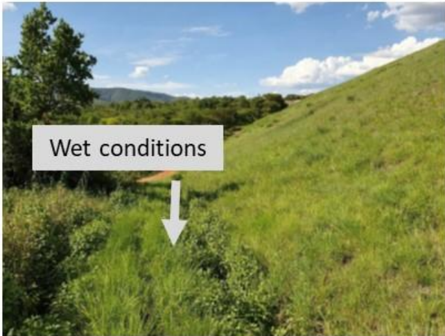
Figure 5: Downstream toe on lower left flank (19 November 2019). Note wet conditions which could be attributed to high phreatic surface within embankment.
