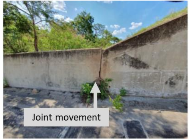
Figure 4: Spillway right training wall joint movement likely caused by tree roots (19 November 2019).
