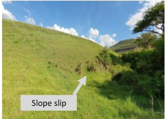
Figure 6: Downstream face of breaching section (fuseplug embankment) on right flank showing local slip (19 November 2019).
