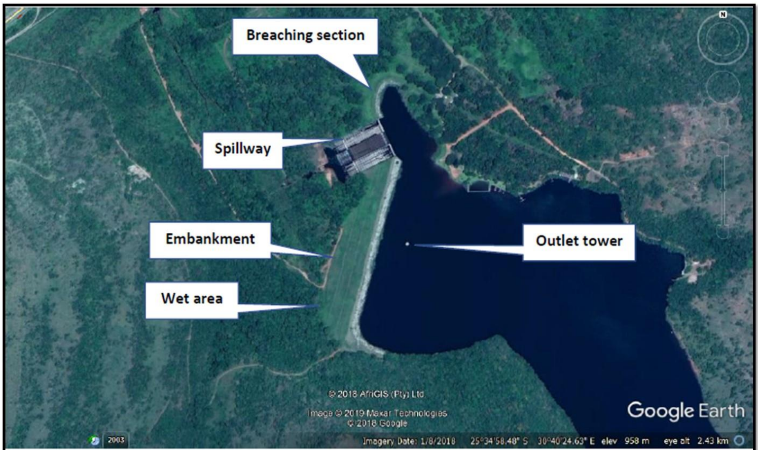
Figure 1: The existing Ngodwana Dam and associated elements (Hagen, 2019).
