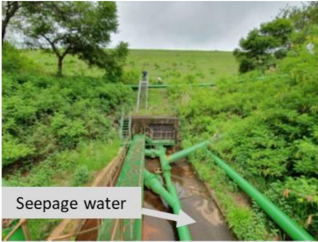
Figure 3: Outlet conduit exit at embankment toe (20 November 2019). Seepage was noted emanating from sides of conduit monitored at v-notch weirs.
