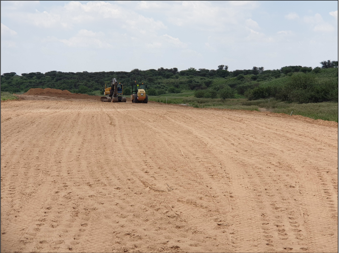
FIGURE 6: CONSTRUCTION ACTIVITY IN THE GA-MOGARA RIVER
