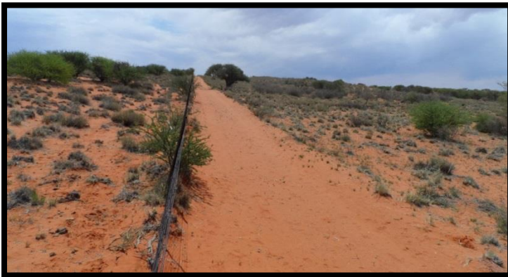
Photo 10: Typical fire protection along boundary fence (Neighbouring property)
