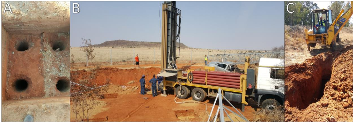
Figure 1-1: A: Piled hole, B: Piling equipment and C: Traditional excavation.
