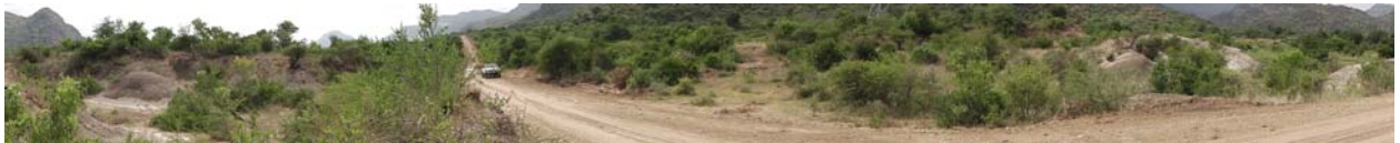
Figure 78: General view showing severe erosion around the river.
