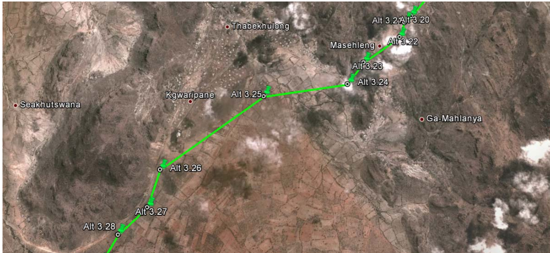
Figure 85: Aerial view of the sector – note land use and erosion.
