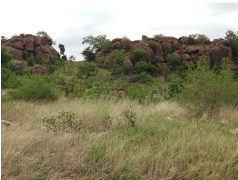
Figure 29: Point near crest where the power line will cross over the mountain.
