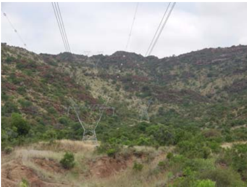
Figure 27: Route crossing the mountain – following the existing power line.
