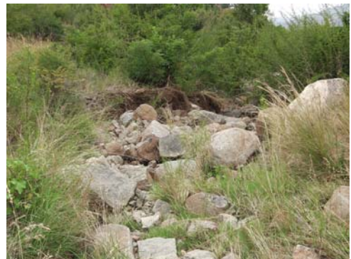
Figure 64: Example of a stream crossing along the corridor.
