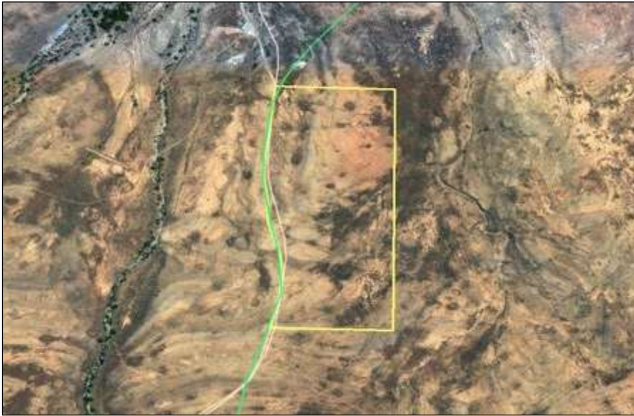
Figure 25: View of the construction site.
