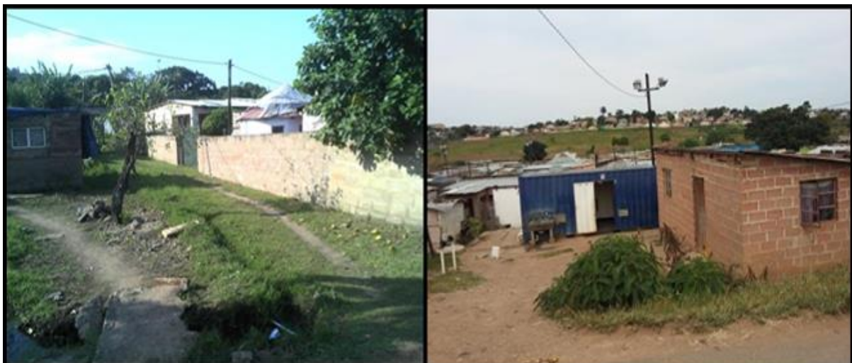
Figure 15: Large scale clearance of natural vegetation has taken place to accommodate the development of formal and informal settlements
