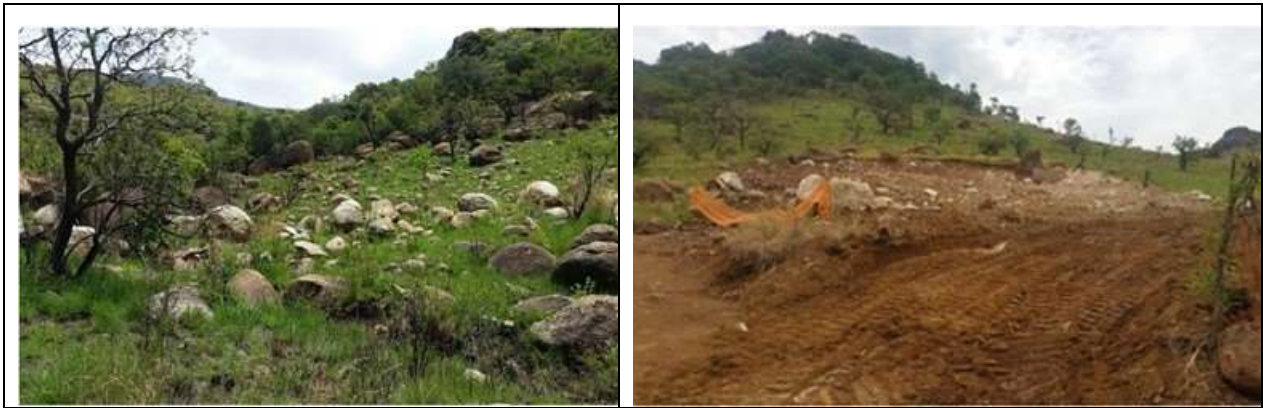
Vent shaft location pre-and during construction
